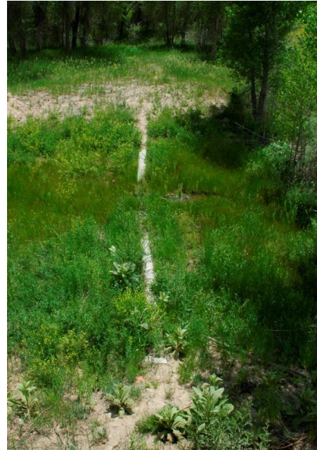
Grade control check structure
