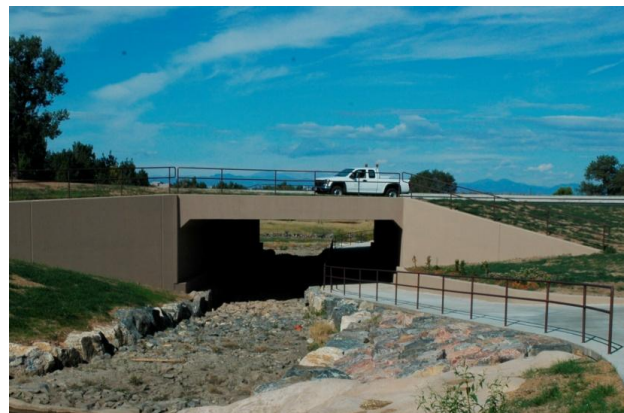
Grade separation using a single span three-sided concrete box culvert.
