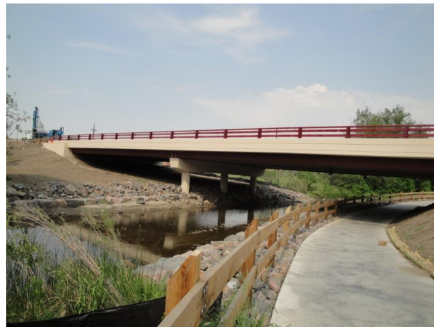
Grade separation at a bridge
