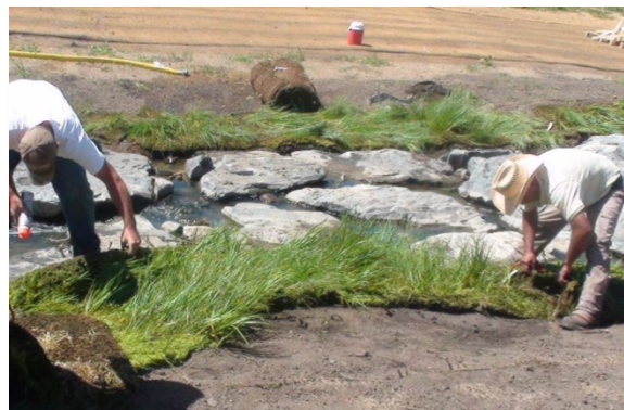
Photograph 13-5. Installation of wetland sod along a reconstructed channel.
