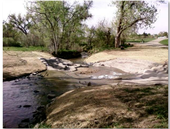
Photograph 13-1. Revegetation in progress in a riparian area along a recently constructed grade control structure. (Photograph courtesy of WWE.)
