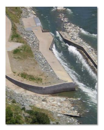
**Photograph 10-33**. The intake works on the American River near Auburn, California relies on a submerged self-cleaning fine screen. The screen is located in the invert of a boatable channel. This design eliminates intake apparatus that can be hazardous to recreationists, screens for fish and solids, and has proven to require relatively little maintenance. Photo courtesy of Placer County Water Agency.
