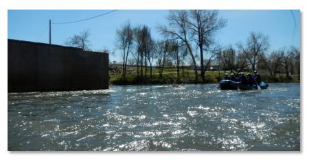
Photograph 10-39. The "pier nose extensions" on this bridge reduce the accumulation of debris and thereby improve safety for in-river users. Photo courtesy of McLaughlin Whitewater Design Group.
