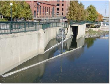
**Photograph 10-32.** The intake at Confluence Park, Denver is located on the side of the river opposite to where the whitewater bypass is located. In addition to this physical separation, buoys, two debris booms and a bar screen were included to help keep recreationalists away from the intake works. Photo courtesy of McLaughlin Whitewater Design Group.
