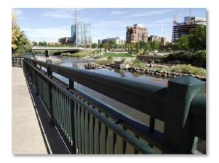
**Photograph 10-8**. At Confluence Park a rub rail was included as part of the rail design. This, in addition to the 14-foot path width, improves safety in this high-use area.
