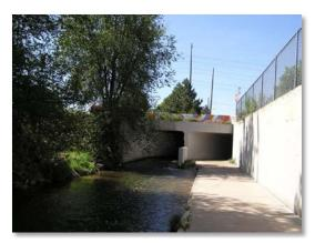
**Photograph 10-16**. Multi-cell culverts can be uninviting, especially if the user is not able to see the other end.
