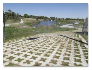
**Photograph 10-26**. Reinforced grass pavement shortly after construction.
