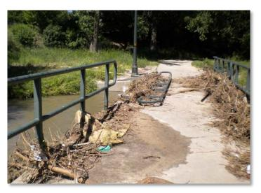
**Photograph 10-5**. Most of the "break-away" rails on this crossing failed to break despite the capacity lost to debris.
