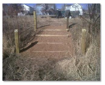
**Photograph 10-24**. Timber steps filled with roadbase are constructed to provide traction approaching a water crossing. Photo courtesy Arapahoe Park and Recreation District.
