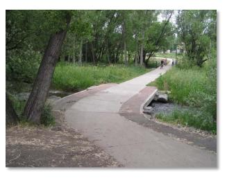
**Photograph 10-21**. A Bear Creek cast-in-place concrete culvert crossing with rumble strips and a crossing with rails in the distance.
