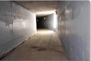
**Photograph 10-18.** A skylight between C-470 travel lanes brings natural light into the Willow Creek path underpass. Note also sediment deposition on path, typical of a long culvert with a mild slope. Photo courtesy City of Lone Tree.
