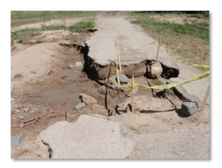
**Photograph 10-11.** A soil cement path approaching a crossing on Sand Creek is undermined on the downstream side due to overtopping. Overtopping protection was not adequate to stop scour damage before losing a section of the path.
