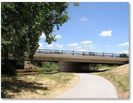
**Photograph 10-14**. This bridge offers safe passage, providing the user with a view of potentially rising water and the path beyond the structure. Additionally, the slope from the path to the roadway offers the user a passable route to higher ground in case of flash flooding.
