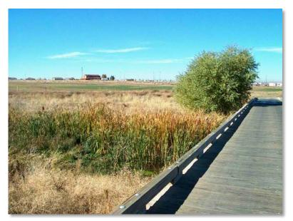
**Photograph 10-6**. Curb rails are typically no higher than 12 inches and can be constructed from a variety of materials.
