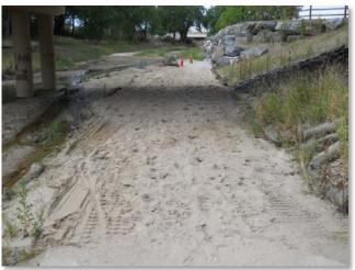
**Photograph 10-2.** Sediment frequently accumulates under crossings. Frequently inundated paths collect sediment and are maintenance-intensive.
