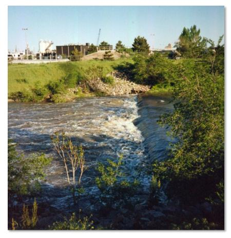
**Photograph 10-34.** Currents downstream of dams or even drop structures can create an overly-retentive hydraulic jump that can trap in-channel users. Sometimes called "keepers" or "drowning machines," these hydraulic conditions can be deceivingly dangerous. The misleadingly dangerous structure shown here created this condition with only 1.5 feet of hydraulic drop before UDFCD retrofitted it to be safely boatable.
