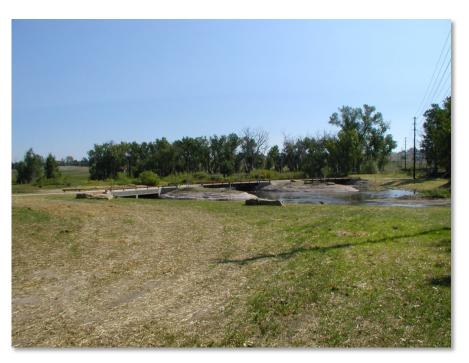
**Photograph 10-20.** This Cherry Creek crossing was split into three segments to accommodate the long span. Curb rails were used and the path was kept low to minimize impediment to flood flows. Photo Courtesy Muller Engineering.
