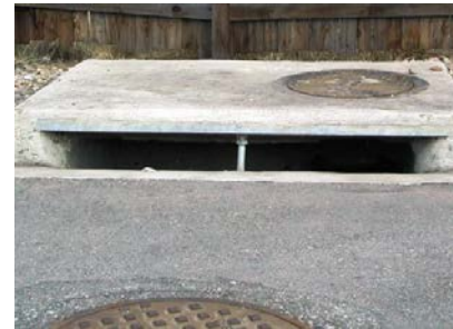
(c) CDOT Type R curb-opening inlet
