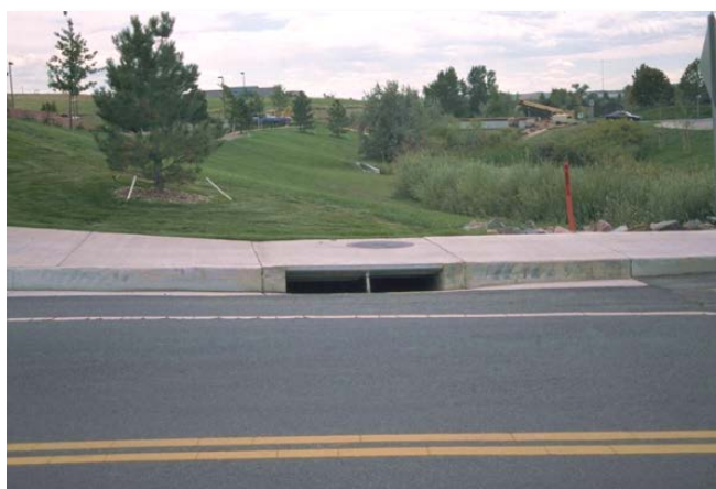
Photograph 7-5. Inlets that are located in street vertical sag curves (sumps) are highly efficient.
