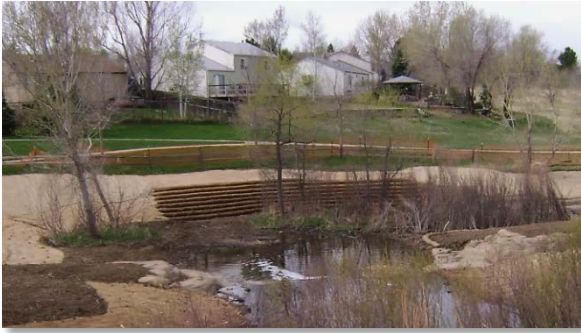
Photograph 8-11. Bioengineering techniques for channel stabilization immediately following construction.
