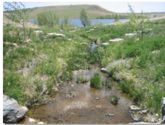
Photograph 8-8. Same channel as photo 8-7 after restoration.
