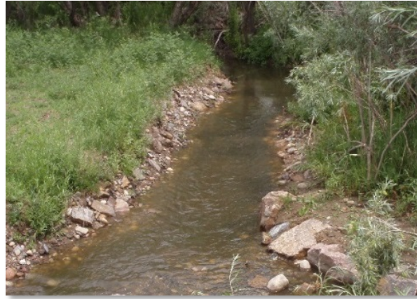
Photograph 8-17. Void-filled riprap used to stabilize the low-flow channel.
