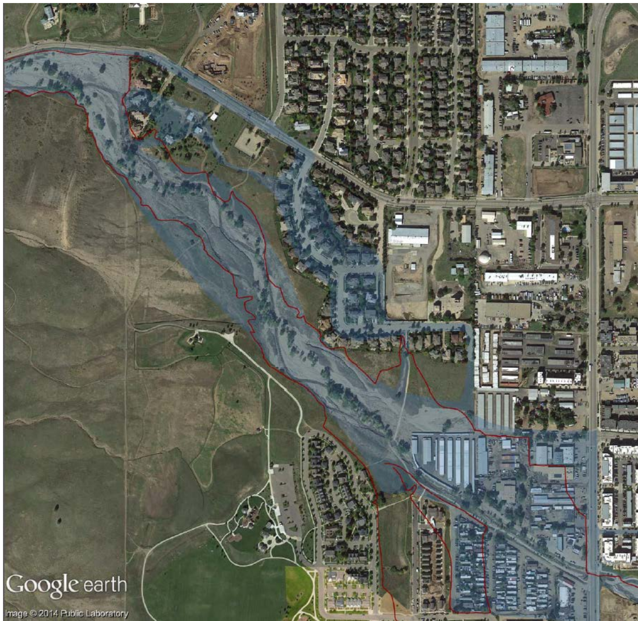
Figure 8-6. Fourmile Canyon Creek, September 2013 flood impacts and floodplain
