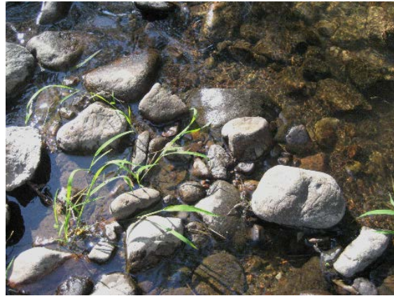
Photograph 8-18. Void-filled riprap is designed to emulate natural rock riffle material; it consists of a mix of rock, gravels, sands, and soil that is densely-packed and able to support riparian vegetation.
