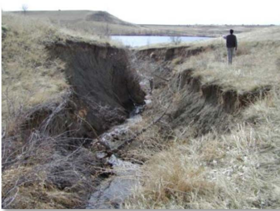
Photograph 8-7. Degraded channel (before restoration).
