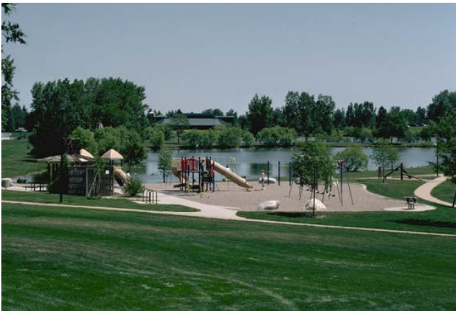
Photograph 3-5. Urban stormwater detention basins can create neighborhood amenities that at the same time serve their flood control function.
