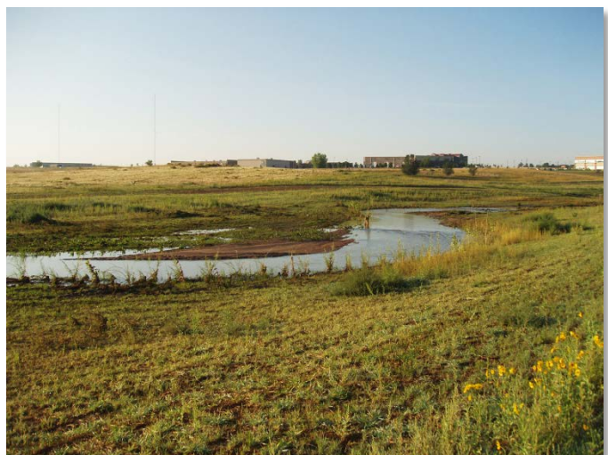
Photograph 8-5. Ample space generally allows softer stream improvements more reliant on cross section shaping and vegetation.
