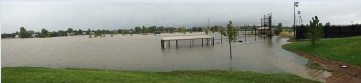
Utah Park providing critical flood detention during the September 2013 flood.
