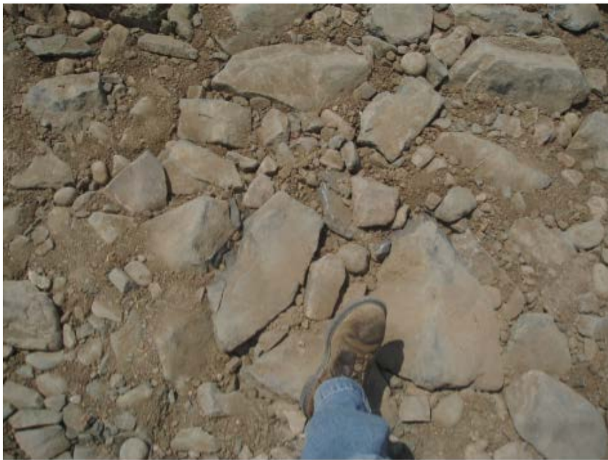
Photograph 8-21. Void-filled riprap after placement and compaction.
