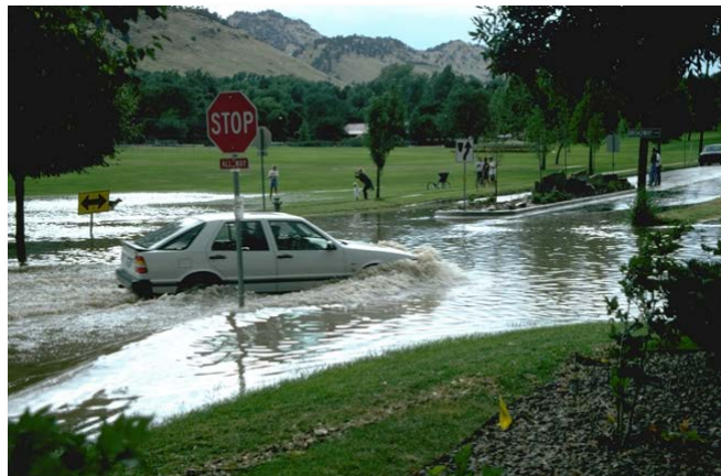
Photograph 3-2. UDFCD drainage criteria are aimed at respecting the needs of safe, unimpeded traffic movement. This intersection represents a long-standing drainage problem needing a solution.
