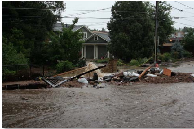
Photograph 6-1. Devastating flooding from Gregory Canyon Creek in Boulder in September 2013 emphasizes the importance of accurate flood flow projections.
