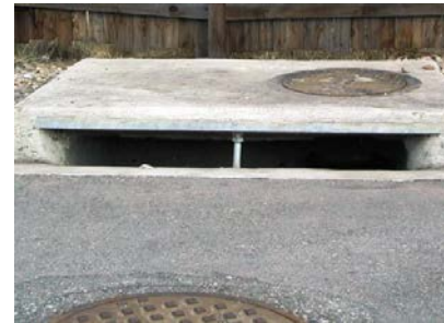
(c) CDOT Type R curb-opening inlet
