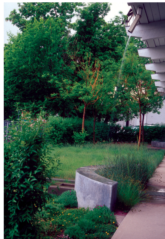
Figure 9. Runoff drains through a spout from the roof of this office building in Denver to a splash block and rain garden below, creating an interesting landscape element while promoting infiltration.
