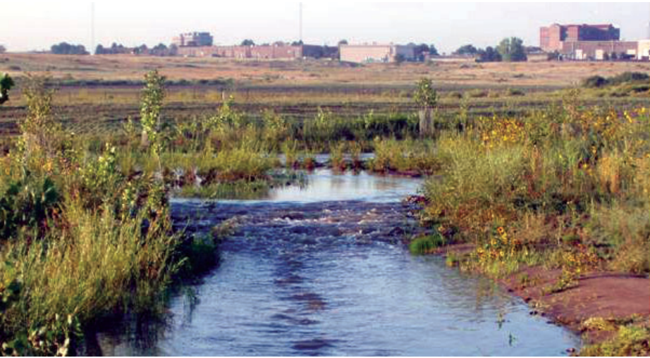
Figure 6. The project's grade-control structures were designed to emulate natural stream riffles using a mix of rock observed in a nearby creek.
