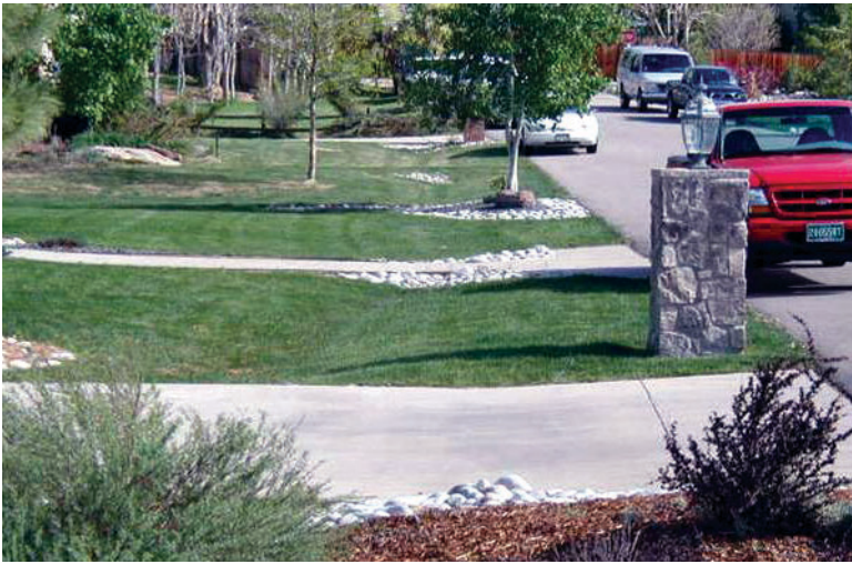
Figures 10 and 11. Grass swales in residential and commercial areas are viable substitutes for inlets and storm sewers, slowing flows and enhancing infiltration and treatment of runoff.
