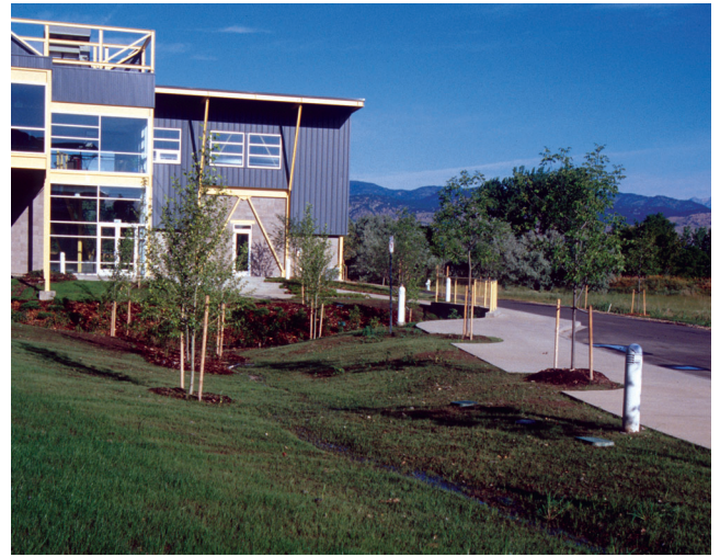
Figures 10 and 11. Grass swales in residential and commercial areas are viable substitutes for inlets and storm sewers, slowing flows and enhancing infiltration and treatment of runoff.
