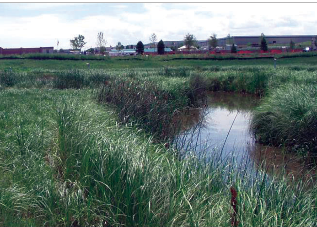
Figure 3. Emulation of natural processes -a design goal for this constructed wetlands detention basin in Greenwood Village, Colorado—allows stormwater management facilities to be functional, cost-effective, and attractive to people and wildlife.
