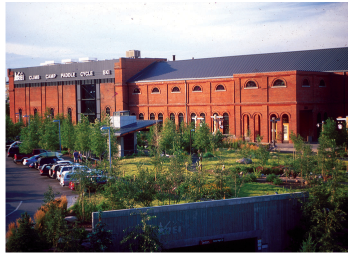
Figure 8. Green roofs, like this garden area over a parking garage in Denver, Colorado, allows rainfall to infiltrate, reducing surface runoff and pollutant loading.
