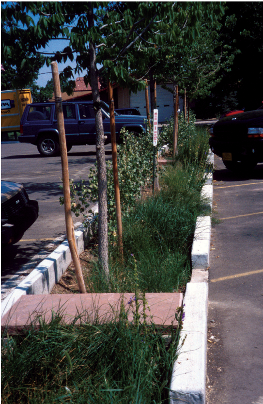
Figures 14 and 15. Parking lot medians and islands provide opportunities to capture runoff from paved surfaces and allow it to infiltrate through planted sandy soil material, a BMP termed bio-retention or porous landscaping detention.
