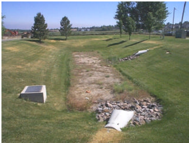
Figure 7. Example of a SFB that functioned well for 10-years in Littleton, CO; was removed by RTD in 1999 to make way for park-and-ride lot expansion.
