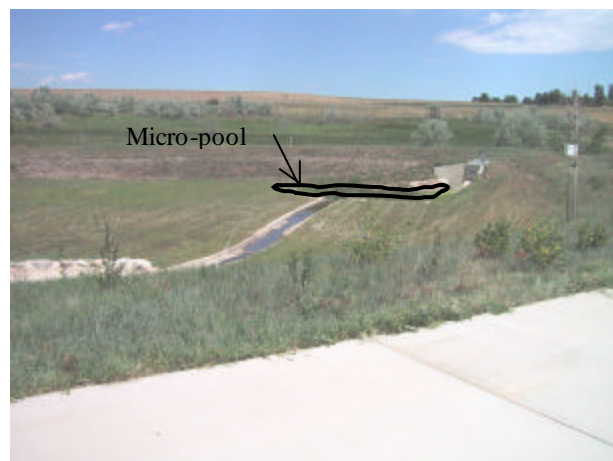
Figure 8. A properly designed EDB in Jefferson County, CO. Note the small wet area (micro-pool) at the outlet during in 2002.
