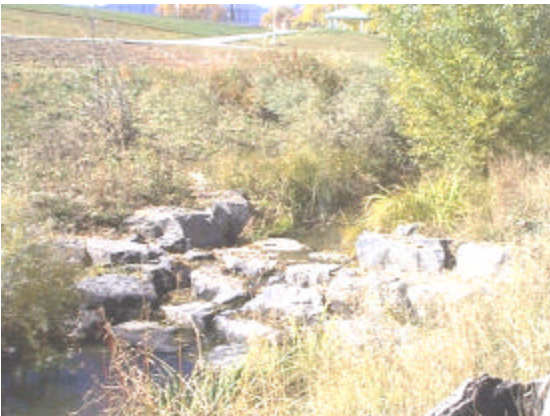
Figure 4. Grade control and soil-riprap stabilized bank - Rock Creek, Superior, Colorado.
