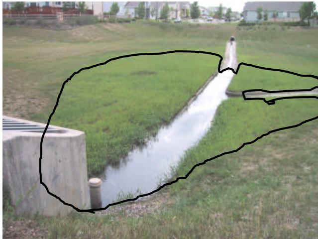
Figure 9. An EDB without a micro-pool. Note the large saturated wet area during a dry weather period in 2002, a drought year, that provides good habitat for mosquito breeding.
