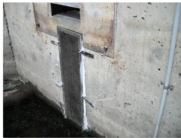
Photograph OS-3. Trash rack after repair.
