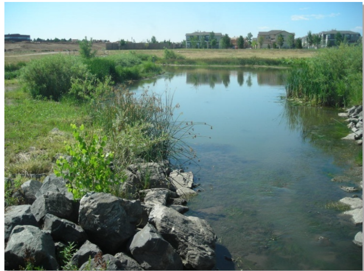
Photograph RP-1. Retention ponds treat stormwater through sedimentation and biological processes including uptake.
