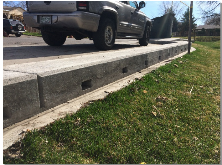
Photograph RR-1. Disconnecting impervious areas and distributing runoff over grass buffers and swales reduces runoff volume and downstream treatment requirements.
