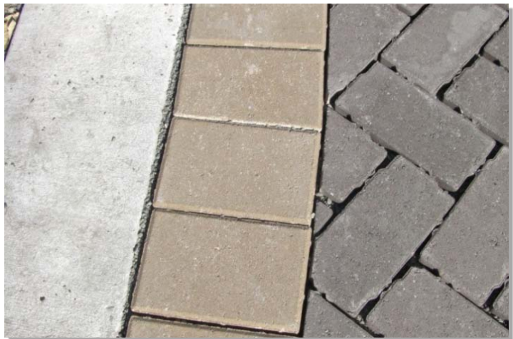
Photograph PICP-2. The very small cut paver shown in this photo could have been eliminated by rotating the paver above it 90 degrees
