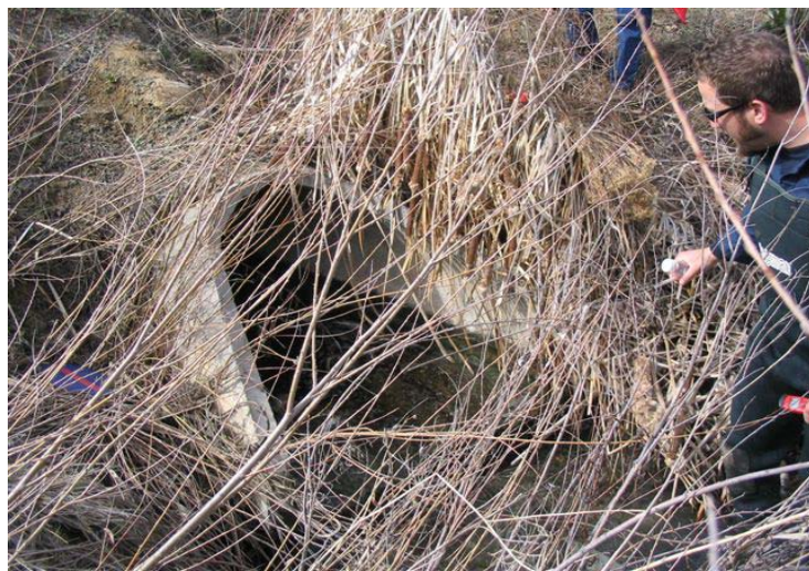
Photograph IDC-1. Mapping and dry weather investigation of storm sewer outfalls is an important tool in identifying and removing illicit connections. Photo courtesy of WWE.
