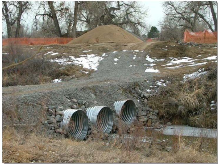
Photograph TSC-1. A temporary stream crossing using culverts. Photo courtesy of Tom Gore.
