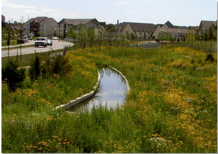
Photograph GB-3. This level spreader includes the added benefit of a sedimentation basin prior to even distribution of concentrated flows from the roadway into the grass buffer. Photo courtesy of Bill Wenk.
