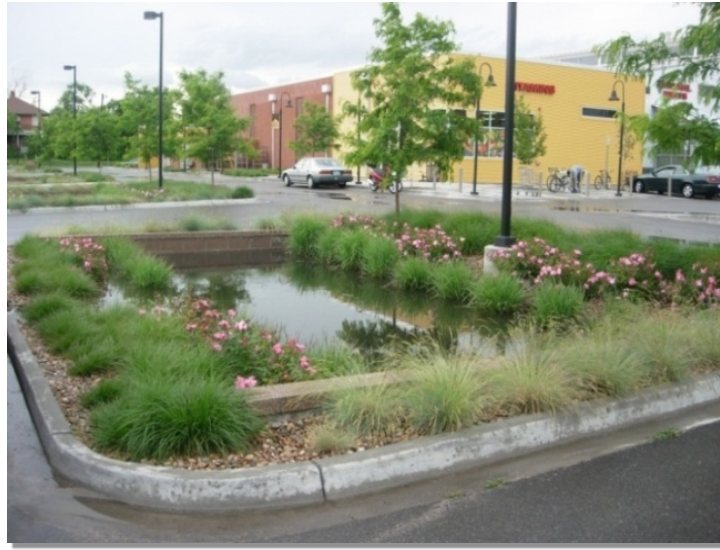
Photograph EDB-4. A series of landscape islands connected by culverts provide water quality and flood control for this site.
