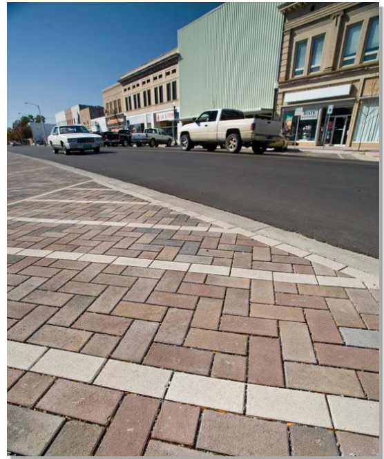
Photograph PICP-1. PICP in downtown Ft. Morgan, CO. Photo courtesy of SEH and the City of Ft. Morgan.
