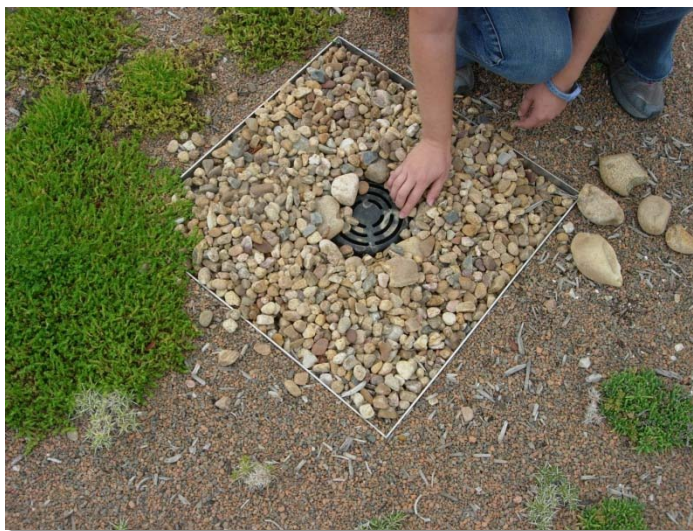
Photograph 6-3. When inspecting roof drains, remove any surrounding rock as well as the inlet grate and visually inspect the drainpipe to ensure it is free of any extraneous materials.
