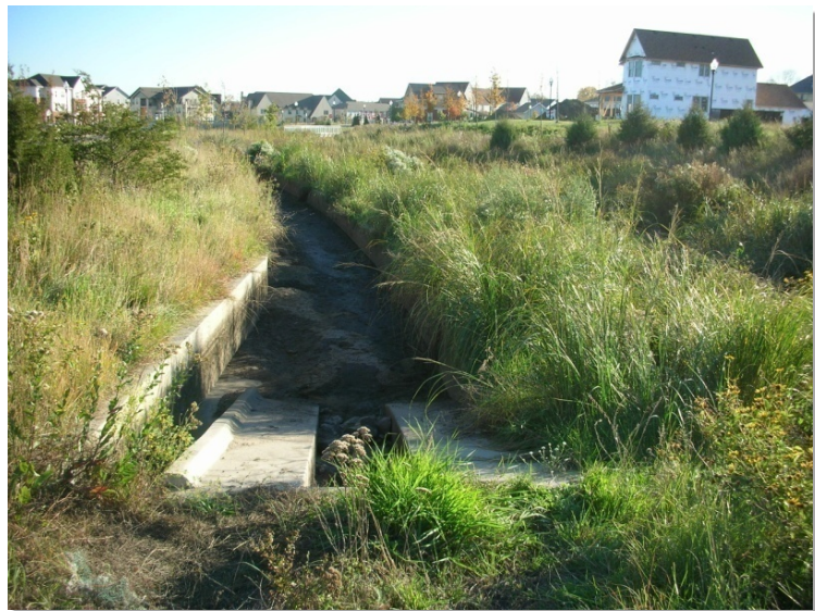
Photograph GB-4. Maintenance access is provided via the ramp located at the end of the basin. Photo courtesy of Bill Wenk.
