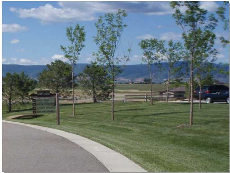
Photograph GB-1. A flush curb allows roadway runoff to sheet flow through the grass buffer. Flows are then further treated by the grass swale. Photo courtesy of Muller Engineering.
