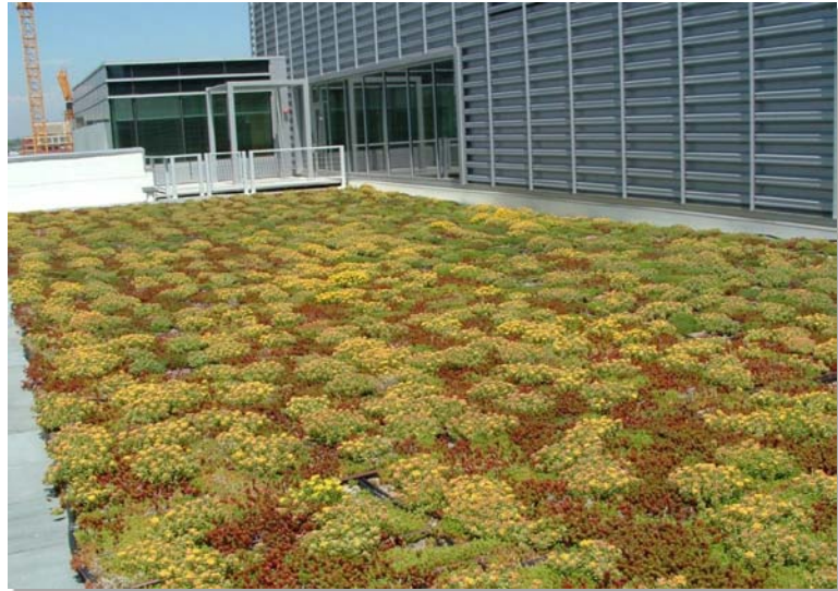
Photograph GR- 4: A modular, extensive green roof in the spring on the Environmental Protection Agency Region 8 Headquarters in downtown Denver. Photo courtesy of Jennifer Boussetol.
