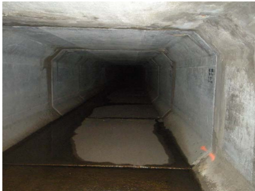
Photo 1 - Alignment and grade looked appropriate
