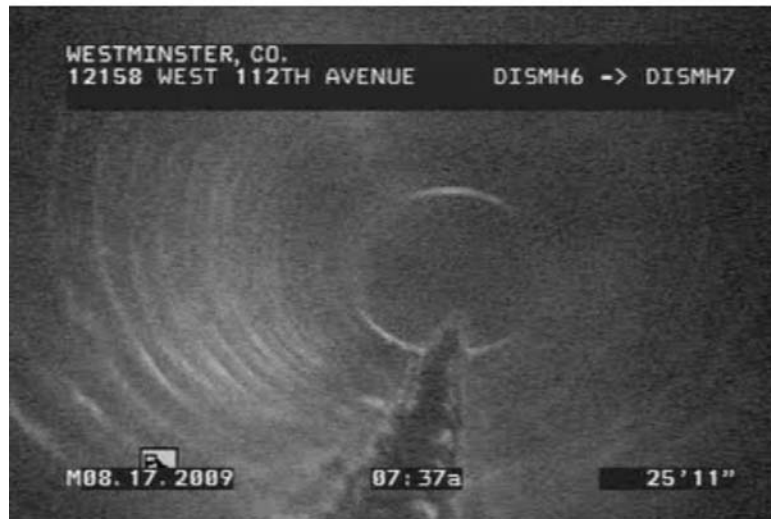
Alignment and grade appear acceptable
