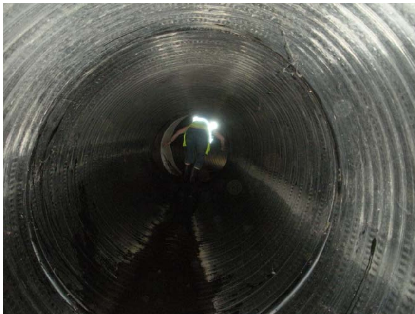
Photo 2 - Pipe alignment, grade, and roundness looked acceptable
