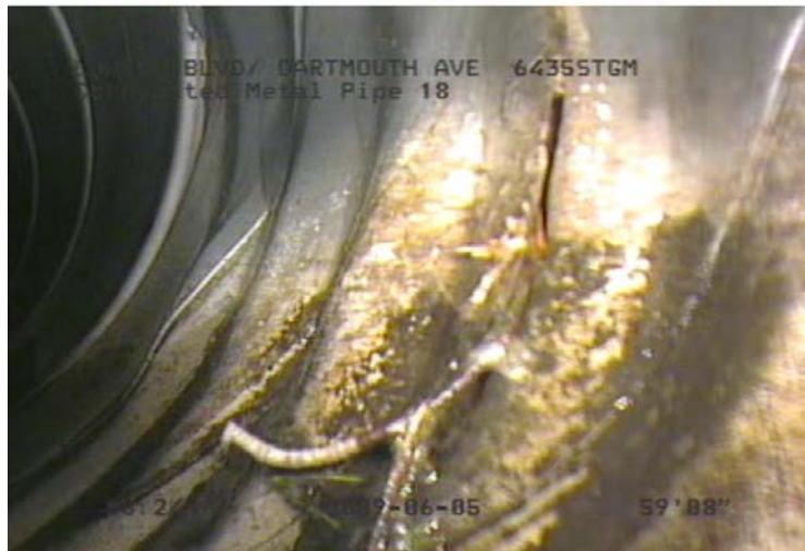
Another damaged pipe
