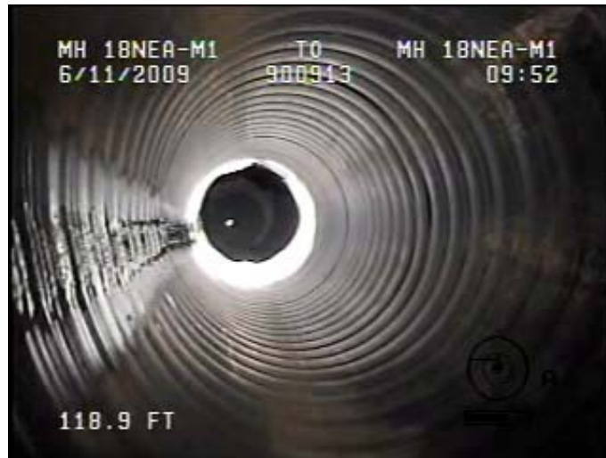
No sedimentation was noticed along the bottom of the pipe
