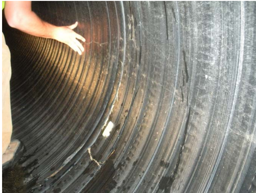
Photo 4 - Joints looked tight and there was no evidence of infiltration
