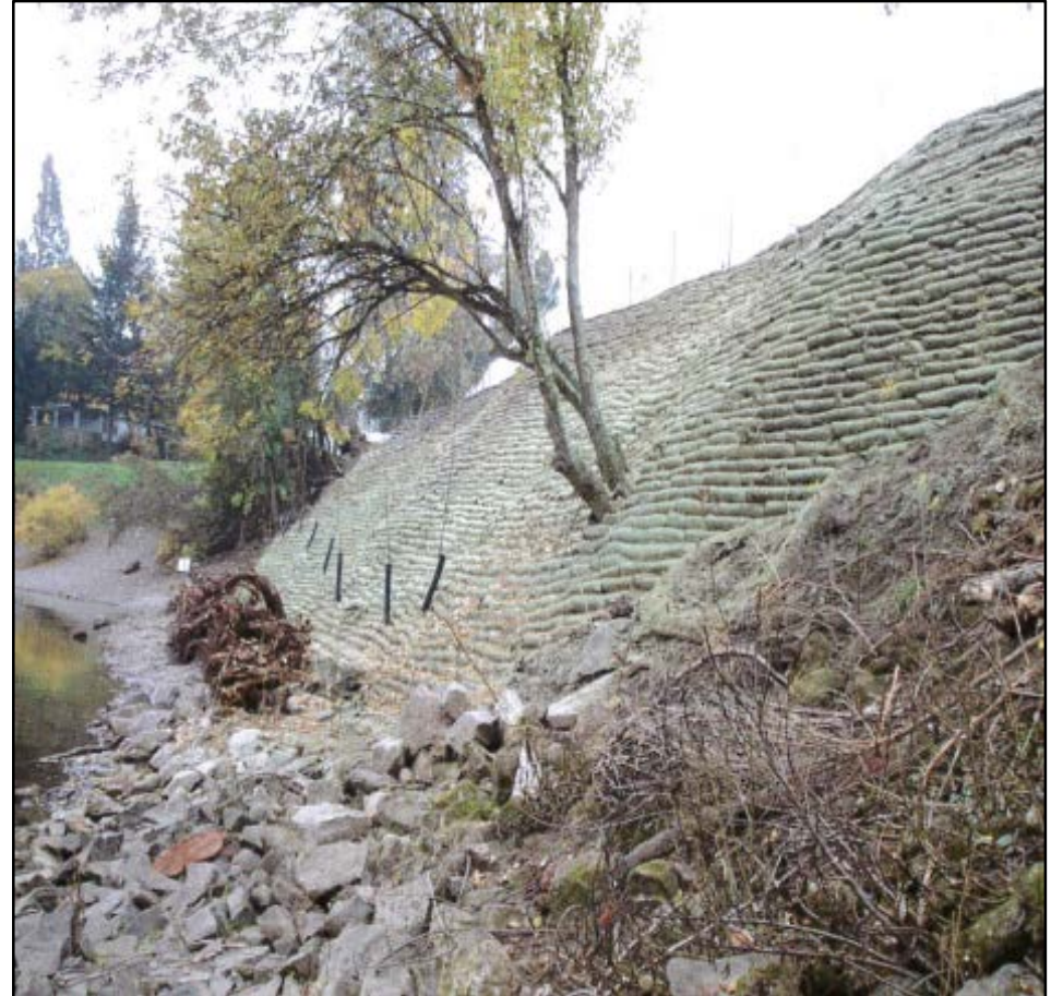
Contaminated Soils Containment
