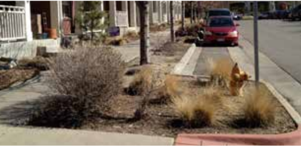
Bumpout Stormwater Planter
