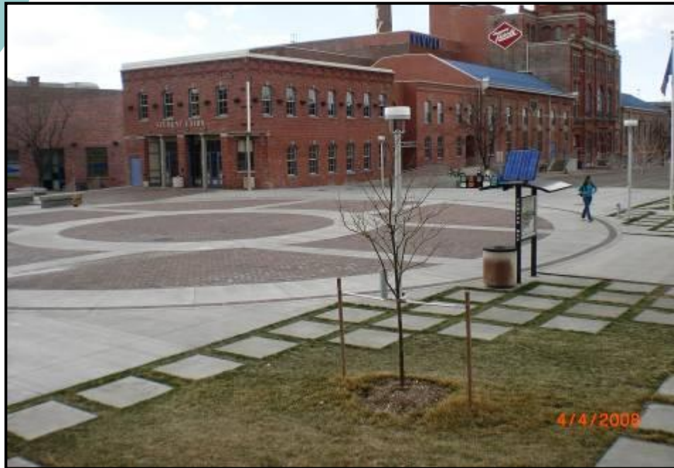
Porous Pavements in UC-Denver Campus
