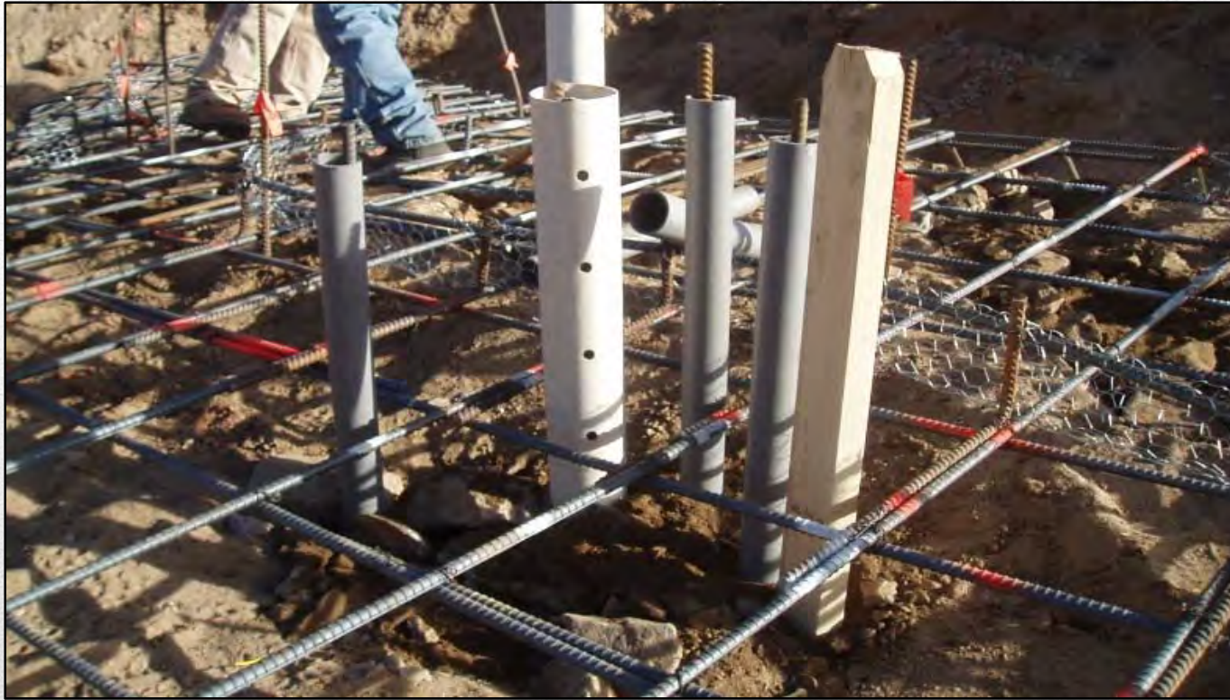
Form Pockets in Concrete
