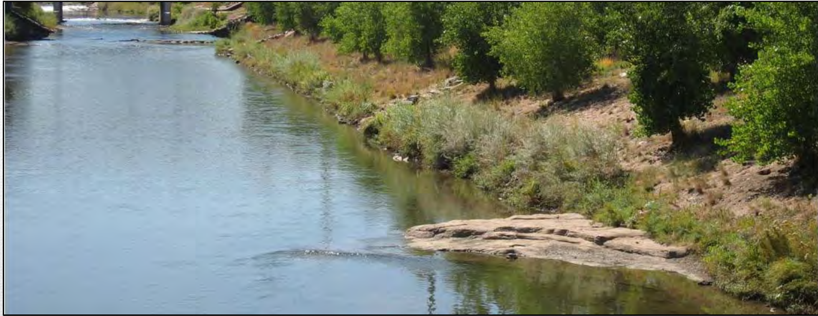
Sculpted Concrete Jetty
