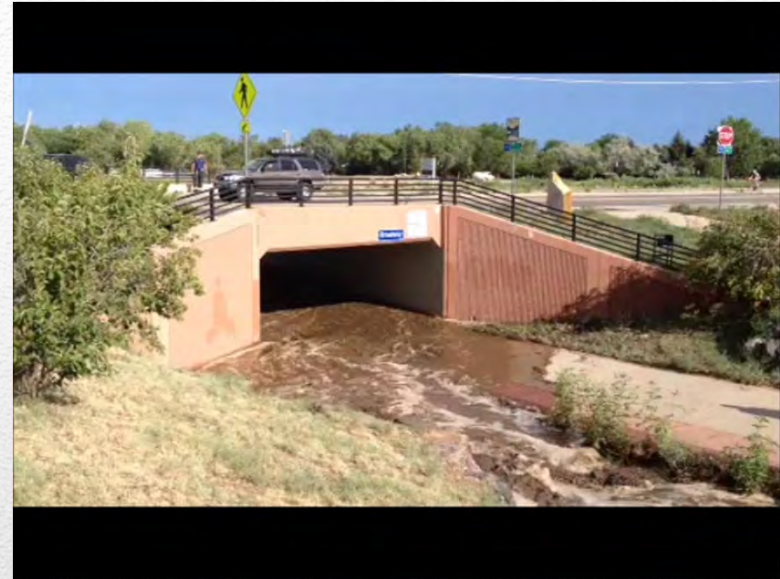
July 30, 2011 Fourmile Canyon Creek at Broadway, Boulder
