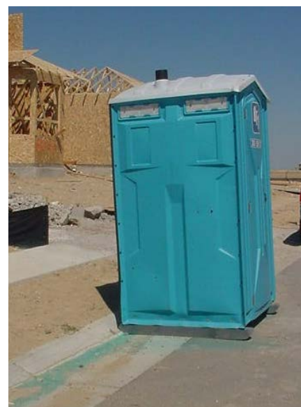
Improperly placed portable toilet with biocide running down gutter toward storm drain. (Photo courtesy of Wright Water Engineers.)
