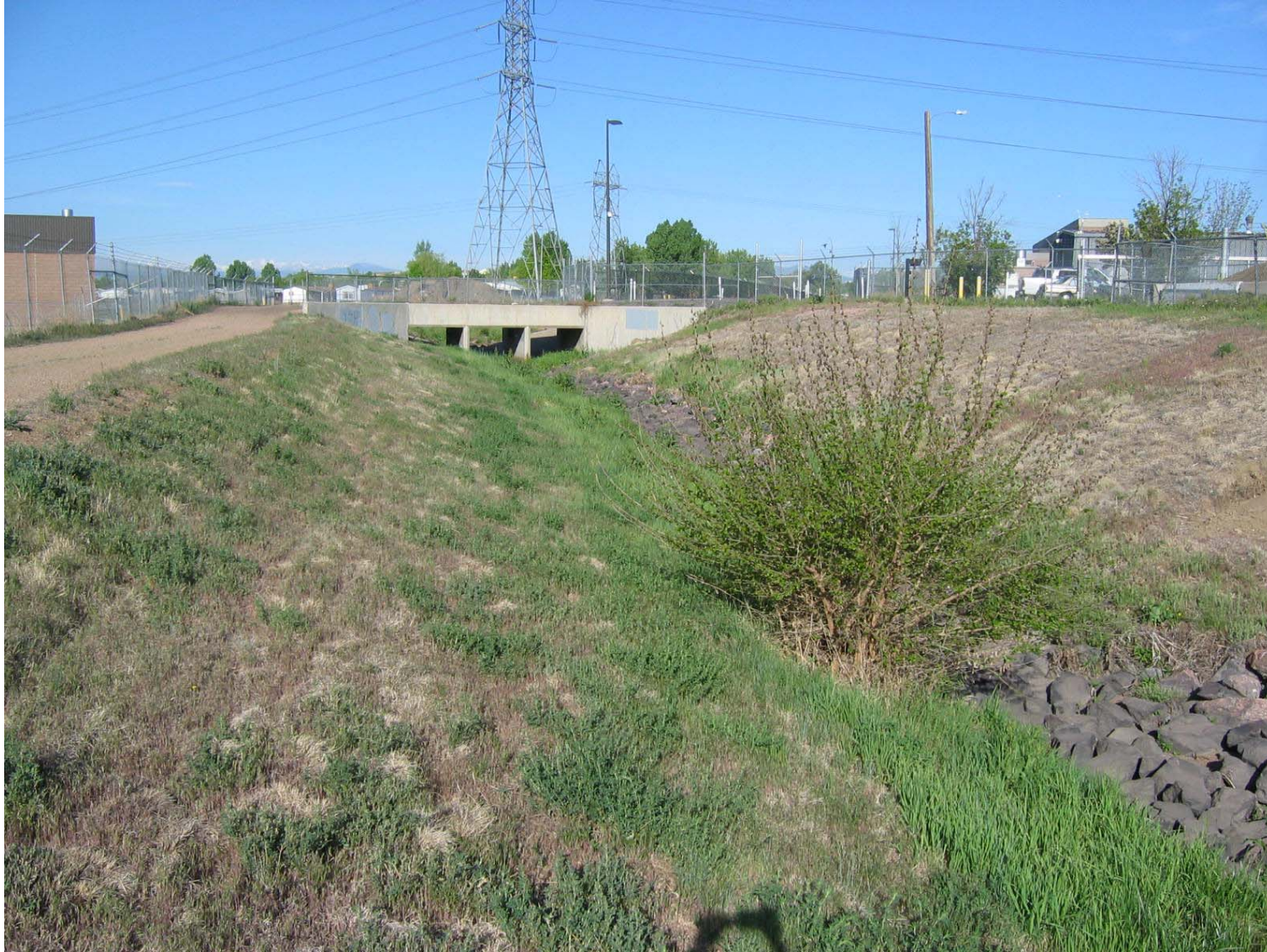
Segment 115 – Devonshire Road to South Platte River Manning's n=0.04
