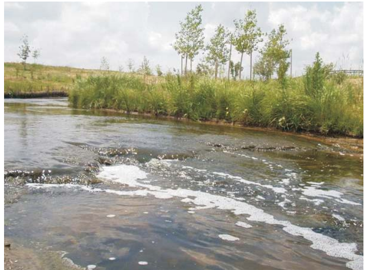
Low flow channel with riffles of shale stone
