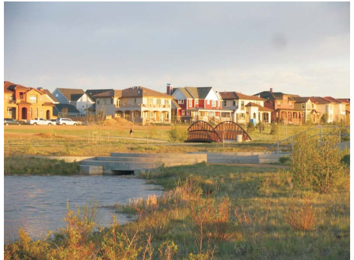
Sculptural detention facility forebay
