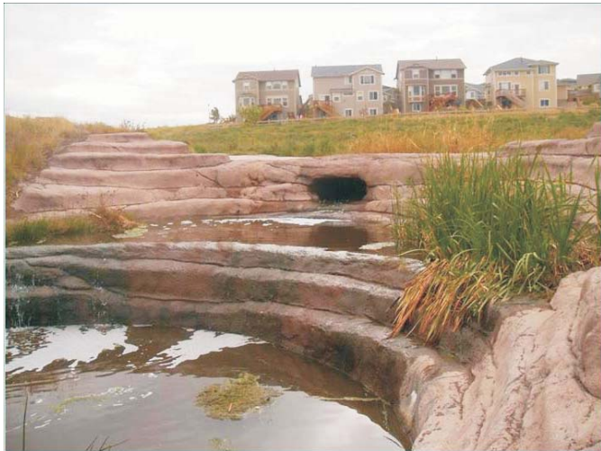
Sculpted concrete drop structure
