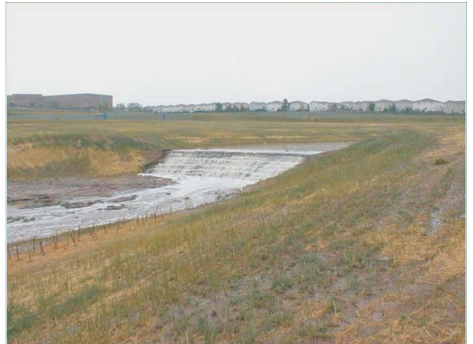
Soil cement drop structure
