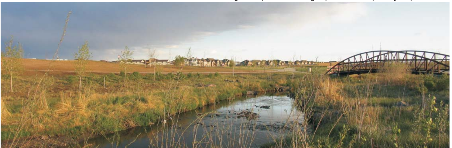
View of low flow channel stabilized with bio-logs and wetland sod
