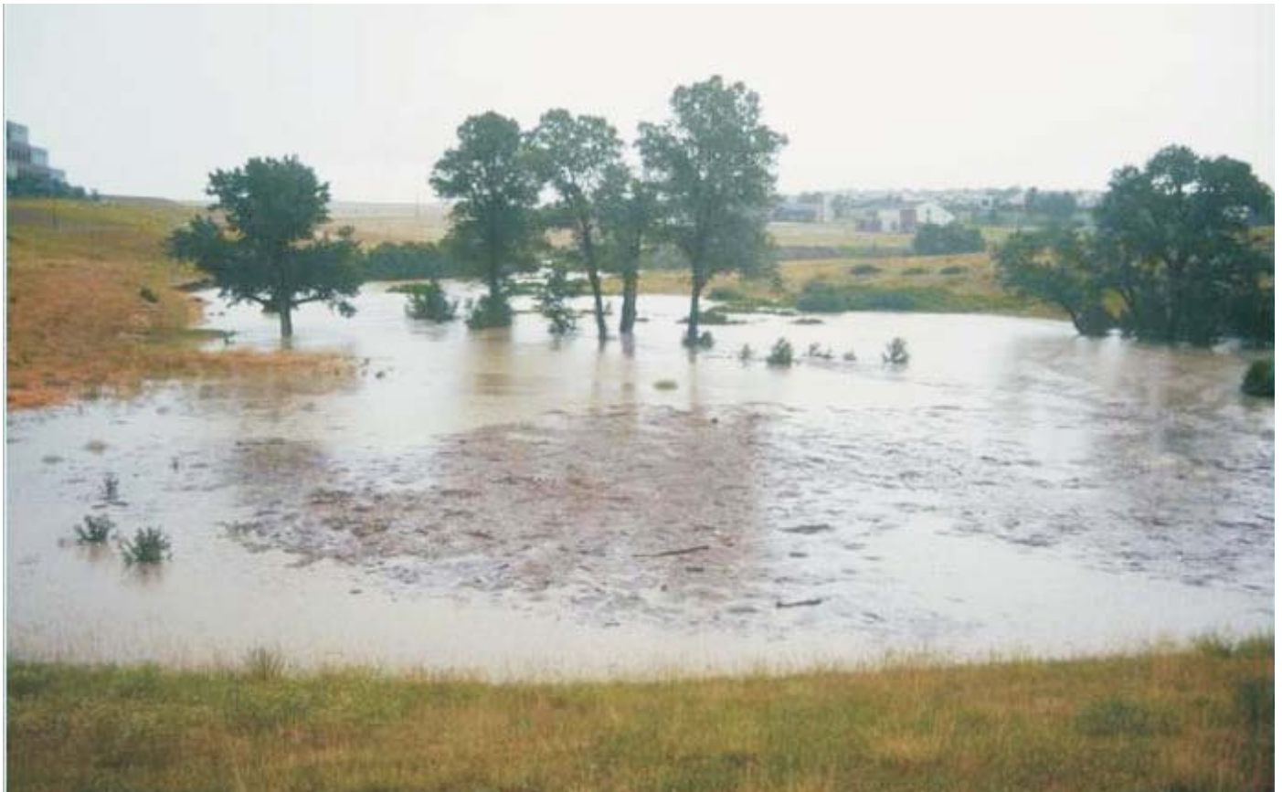
Broad floodplain illustrates it can accommodate large storm events without compromising residential units
