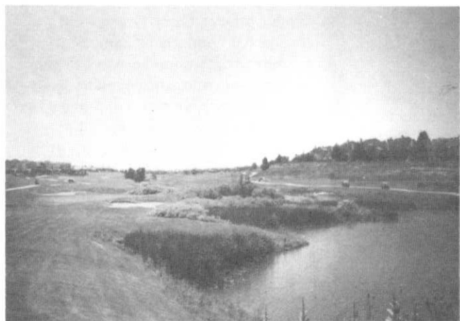
Figure 3. Cook Creek after construction of the grade control structures.
