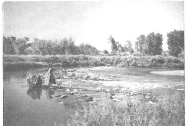
Figure 7. South Platte River grade control structure.
