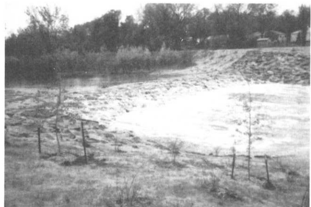
A Grouted Sloping Boulder Drop Structure on Cherry Creek in Denver constructed by the Maintenance Program.
