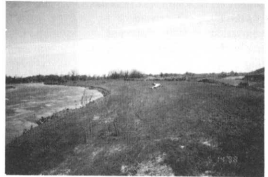
Before and after views of Suburban Sand and Gravel Co-op project. Note the gravel pit on the right side of the berm.
