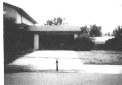
July 25, 1998 high water debris line at 918 E. 7 th Ave.
