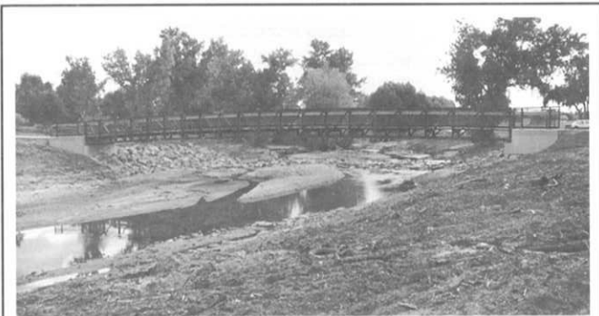
Drop structure and pedestrian bridge across Cherry Creek in Arapahoe County.
