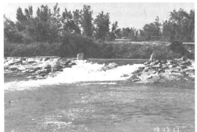
C470 utility crossing before and after.
