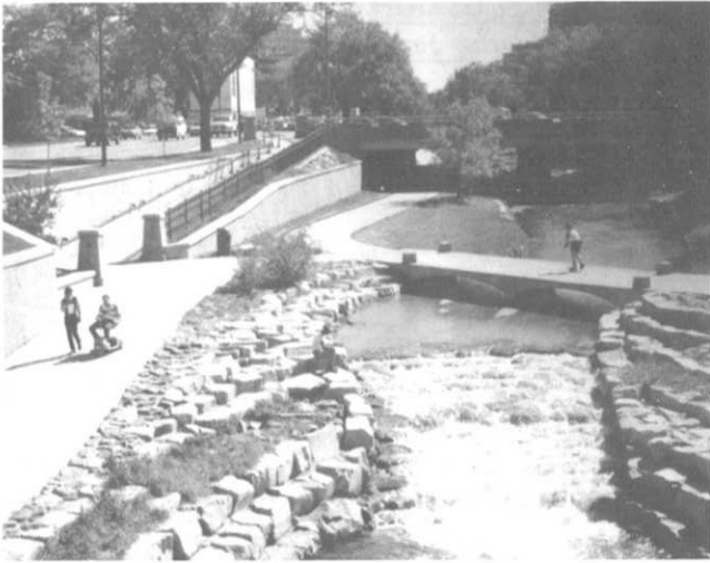
The GSB can be modified for special applications, in this case the Creekfront project on Cherry Creek in downtown Denver. The left picture is looking upstream and the right picture is looking downstream.
