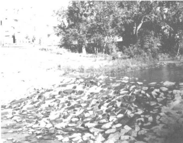
The Maintenance Program uses the GSB for new and replacement drop structures on Cherry Creek downstream from the dam.
