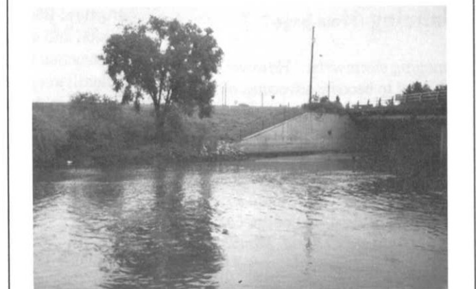
Top: Eighteen foot high retaining wall before site restoration. Bottom: The site was opened up to the river by cutting back the retaining wall and adding railings, all without the loss of any trees.
