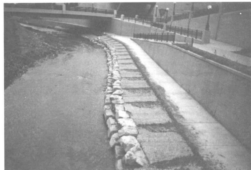
Low flow channel repairs on Cherry Creek near the confluence.
