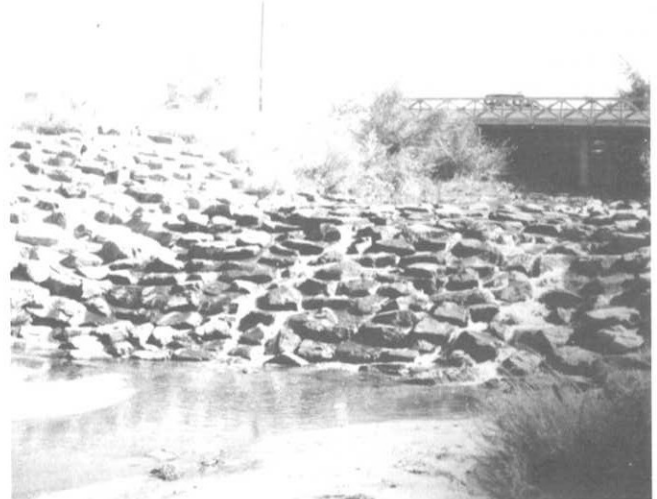
The Maintenance Program uses the GSB for new and replacement drop structures on Cherry Creek downstream from the dam.
