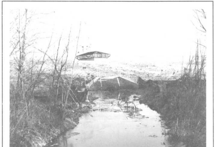
Outlet structures at newly completed Williamette Pond detention facility.
