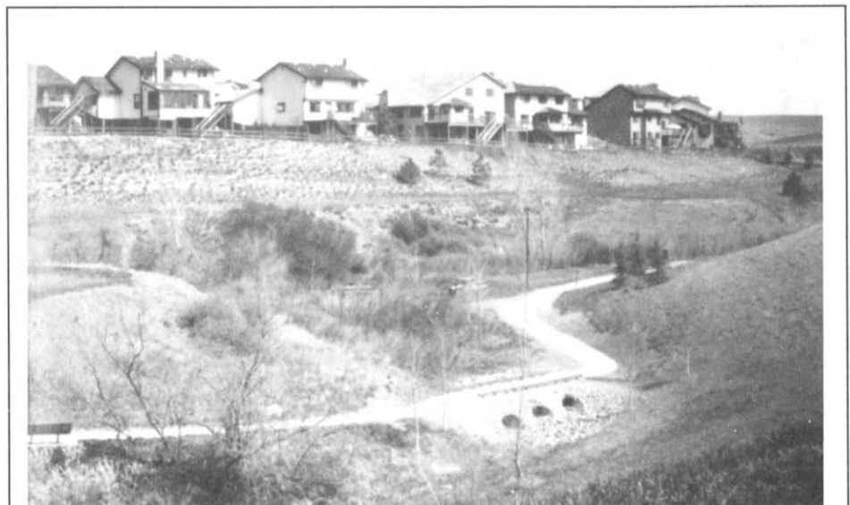
Most people would like to see this kind of treatment of our drainageways, but . . .
