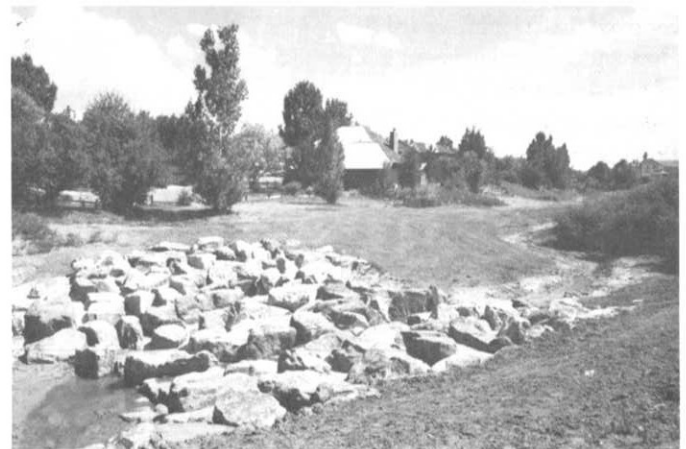
Grade control structure on Spring Creek in Arapahoe Co.
