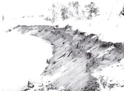
Typical bank erosion damage.
