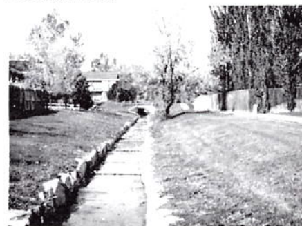
Concrete bottom trickle channel at Middle Branch Hylands Creek.
