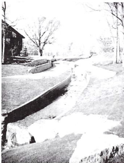
Figure 2. The low flow channel as it existed shortly after construction.
