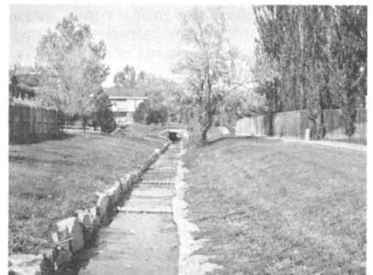
A recently rehabilitated channel in Westminster.
