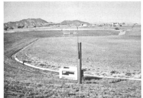
A District rain and stage ALERT gauge at Drainage-way Detention in Louisville.
