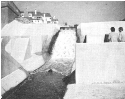
An energy dissipater on Little Dry Creek in Westminster.
