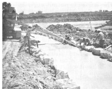
Constructing a low flow channel consisting of concrete bottom and boulder sides at Slaughterhouse Gulch.
