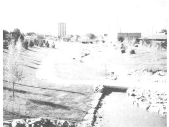
Little Dry Creek construction in Englewood. A grass lined channel with boulder sided trickle channel.
