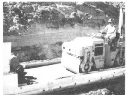
Placing soil cement in Sand Creek.
