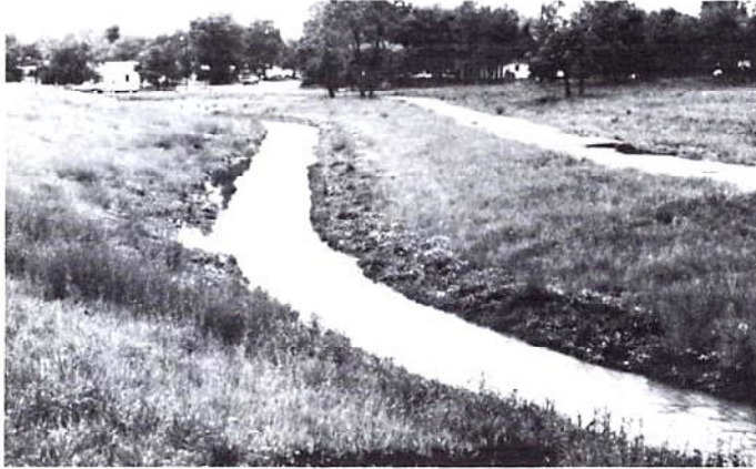
Native grass-lined channel with concrete trickle channel and maintenance trail. This is Sanderson Gulch in Denver.
