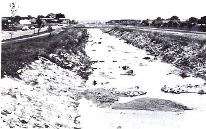
Niver Creek, a riprap lined channel in Adams County.
