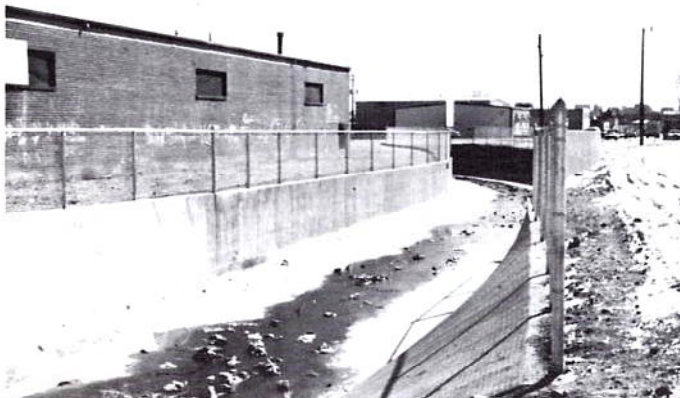
Entrance to Weir Gulch concrete channel in Denver.
