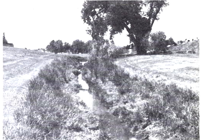
Figure 2—Earth trickle channel on Big Dry Creek in Arapahoe County
