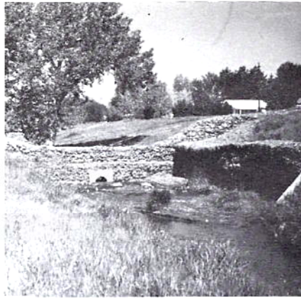
Figure 8—Drop structure on Sanderson Gulch in Denver.
