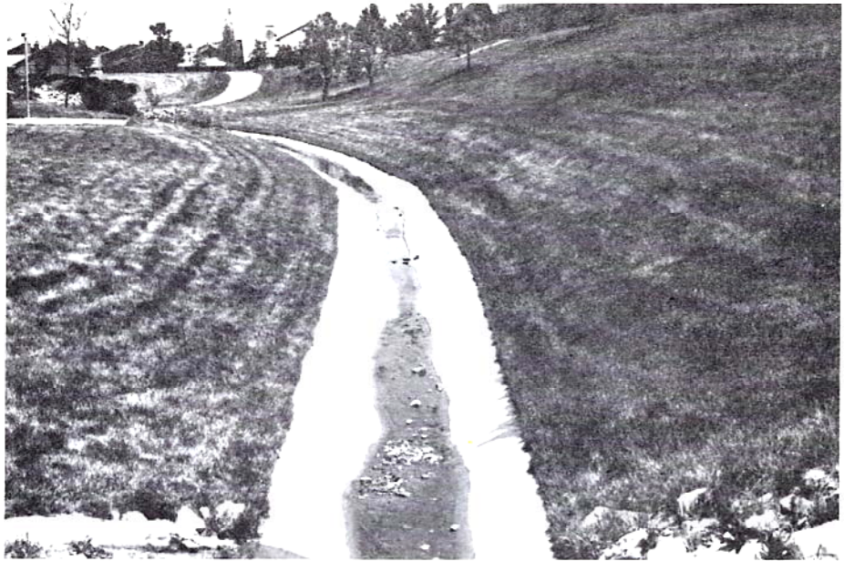
Figure 7—Concrete V-shaped trickle channel on Goldsmith Gulch in Arapahoe County.
