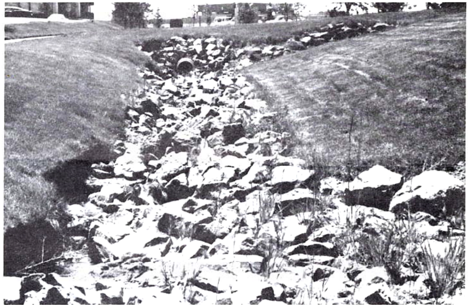
Figure 5—Rocklined trickle channel on Goldsmith Gulch in Arapahoe County.
