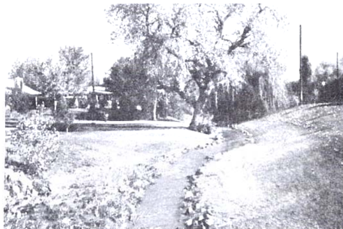
Figure 3—Rocklined trickle channel on Lena Gulch in Wheat Ridge
