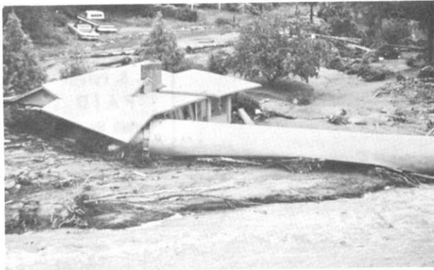
The siphon from Big Thompson Project was washed downstream.
