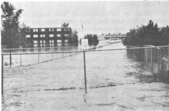
Looking downstream from 19th Avenue
