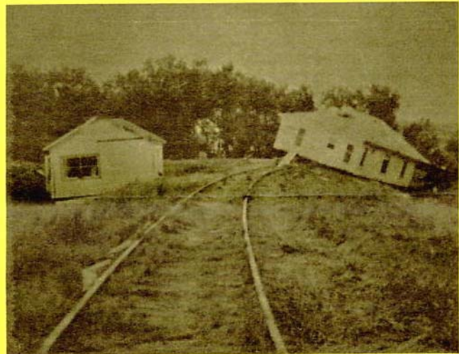
MORE BUILDINGS CARRIED INTACT BY FLOOD WATERS TO NEW SITES
