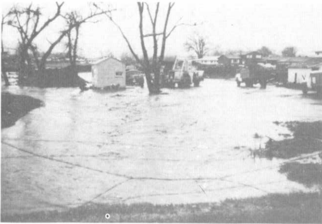
RALSTON CREEK OVERFLOW AT SIMMS STREET DURING MAY 1973 STORM.
