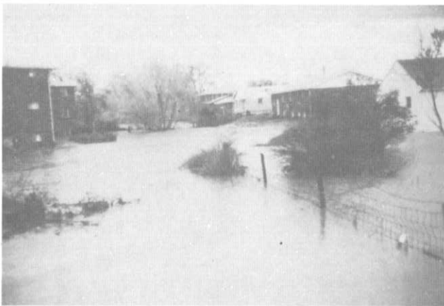
FLOODWATERS FROM RALSTON CREEK IN VICINITY OF WADSWORTH BOULEVARD.
