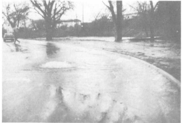
WATER ERUPTING FROM MANHOLES ALONG RALSTON CREEK BELOW CARR STREET.
