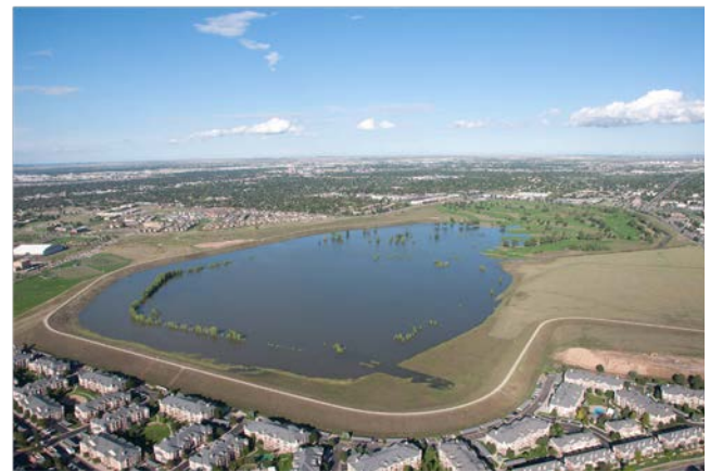
Westerly Creek Dam flood pool two days after the rain
