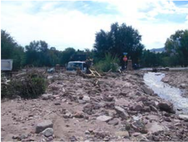
Sediment deposition and post-flood creek alignment (pre-flood alignment is left of photo).
