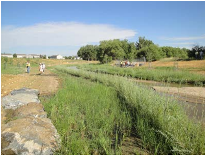
Wetland mats three months after installation.
