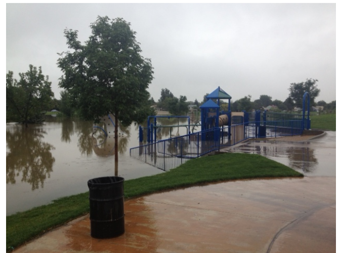
Multipurpose detention facilities have significant social benefits. For example, this park in Aurora features baseball, tennis, soccer, passive recreation and on September 11 th , 135 acre-feet of flood storage.
