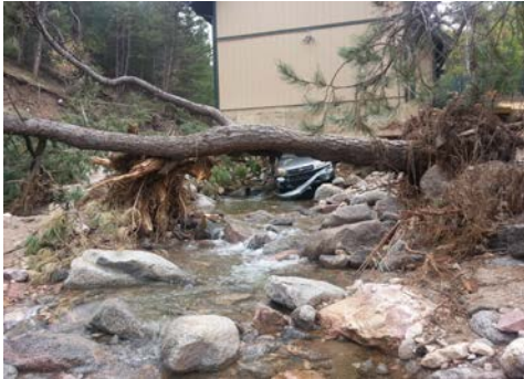
September 2013 flood damage along Fourmile Canyon Creek in Boulder County near UDFCD border.
