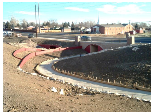
The Grange Hall Creek culvert and underpass after construction.
