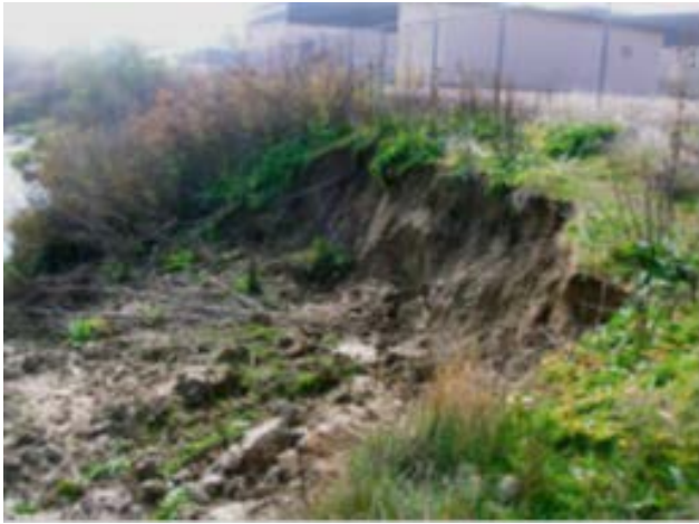
Big Dry Creek erosion at Broomfield WWTP.
