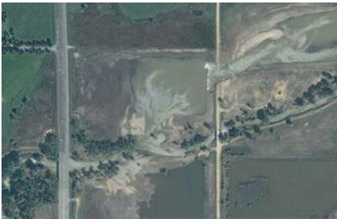
Post-flood aerial photo of Boulder Creek channel migration at 109 th St.
