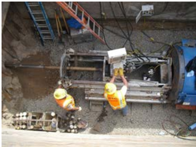
Guide rod installation for trenchless construction of the 60-inch storm sewer.
