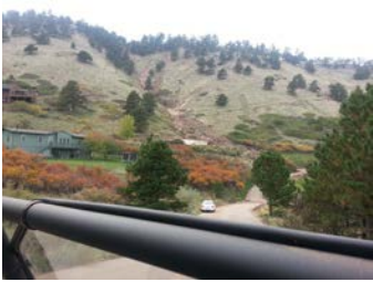
Landslide in Two Mile Canyon in Boulder County.
