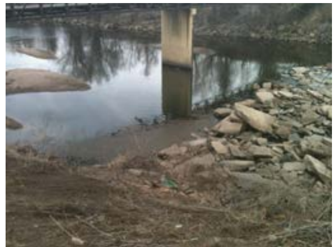
The “informal” grade control structure near the Metro WWTP.
