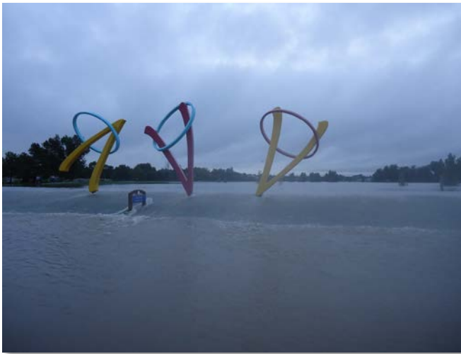
Exposition Park and Regional flood Detention Facility in Aurora, CO; a city park under dry-weather conditions served its dual purpose as a flood storage detention basin during September.
