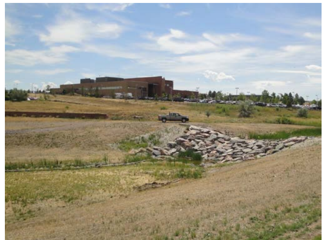
Recently constructed drop structure into Detention Basin L-2.
