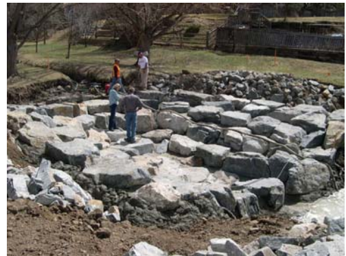
Grouted sloping boulder drop on Greenwood Gulch
