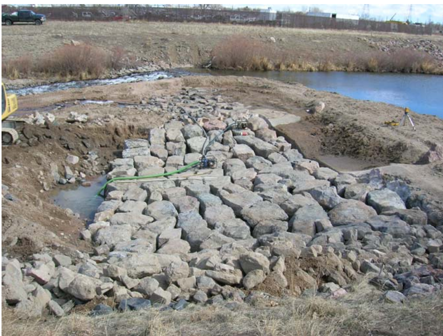
Boat Chute Repair Below Union Ave
