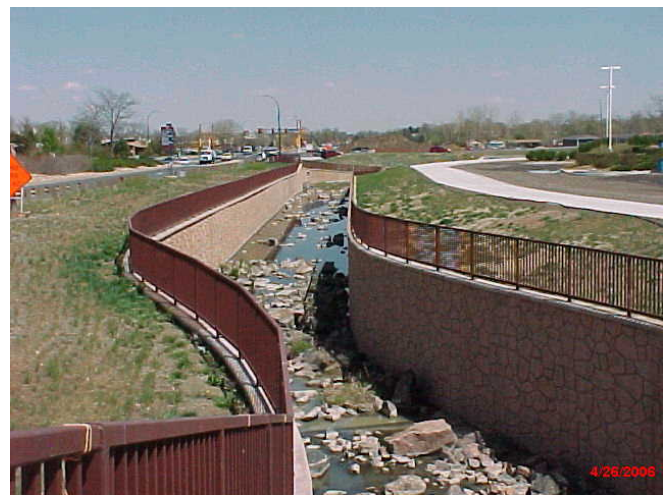
The Van Bibber Creek project was very complex, requiring the use of grass-lined channels, vertical wall channels and a large box culvert.
