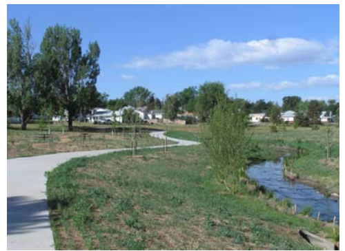
New channel upstream of Florida Avenue
