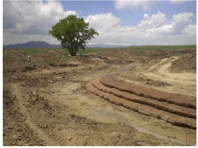
Soil lifts under construction
