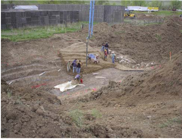
Large Drop Structure being poured
