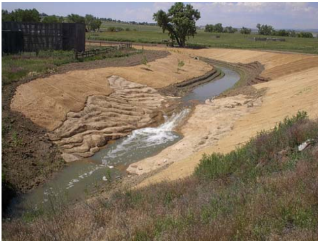
Sculpted concrete drop structure at project completion
