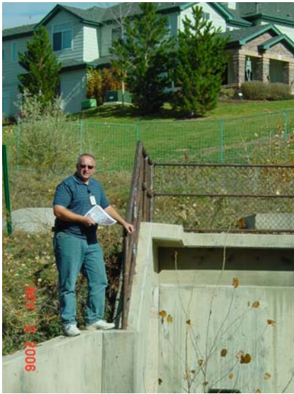
Douglas County inspector Brian Schultz on the hunt for forgotten drainage projects in Highlands Ranch.
