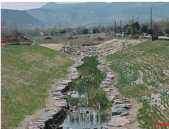
The Van Bibber Creek project was very complex, requiring the use of grass-lined channels, vertical wall channels and a large box culvert.
