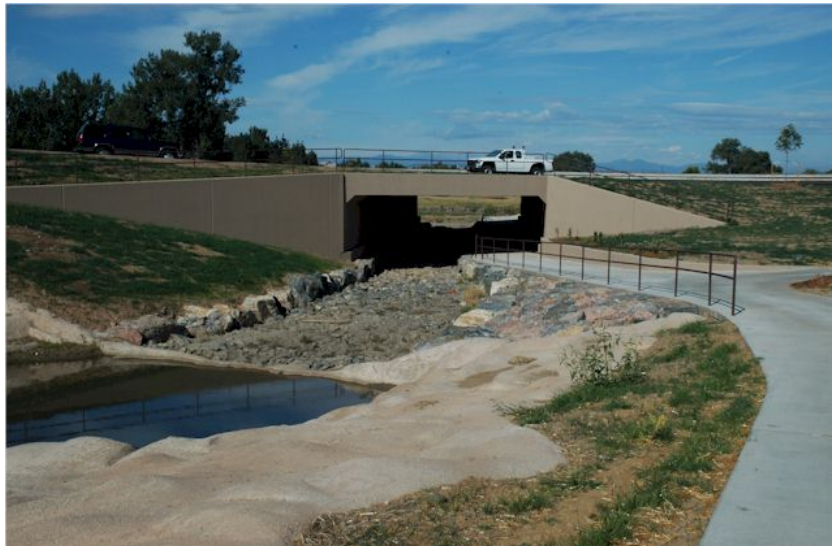
View from the top of the completed drop towards the Twenty Mile Road culvert crossing. Note the grouted boulder transition and open three-sided concrete box culvert section.
