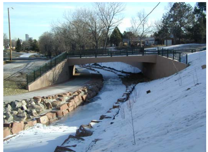
Tennyson Street Bridge at Lakewood Gulch
