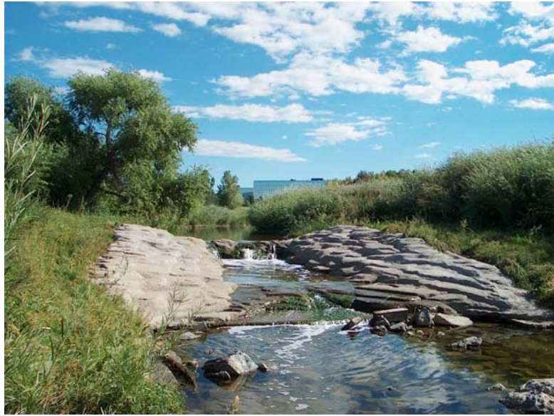
Faux rock drop structure sculpted to resemble rock outcropping.
