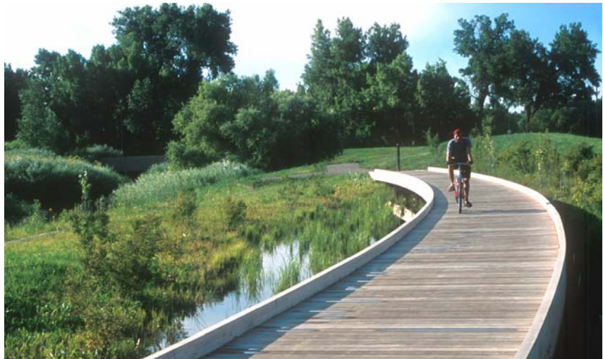
The "floating bridge" over the water quality pond.
