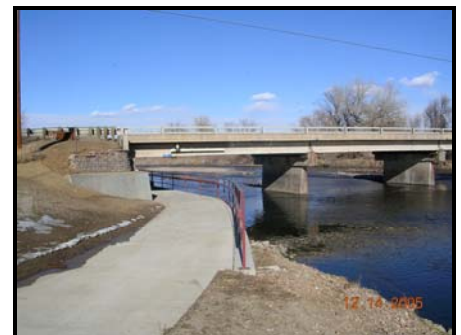
Photo 2: Newly completed 104 th Avenue Trail Underpass
