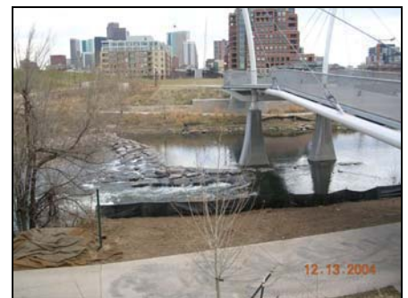
Photo 3: New 16 th Street Pedestrian Bridge and Grouted Boulder Grade Control. Note the fish migration and boater chute along near bank to keep the riverbed from degrading.
