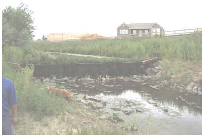
Piney Creek drop structure
