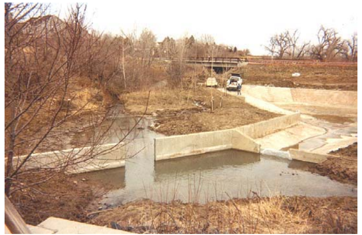
Left: Willow Creek sediment trap at Dry Creek Road. The pond is full with 800 to 1000 cubic yards of sediment. One of our indicators for when it is time to remove the sediment is when people start having picnics on our "beach." Right: The left side of photo shows the Willow Creek channel. The freshly cleaned sediment trap is on the right. The diversion boards are still in place to keep water out of the sediment trap while it is being cleaned.
