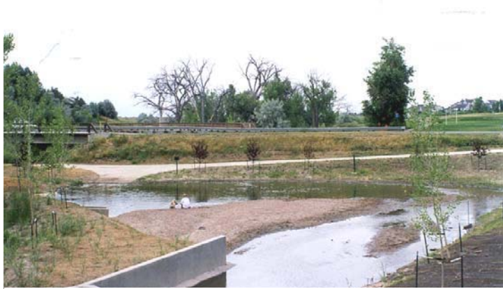
Left: Willow Creek sediment trap at Dry Creek Road. The pond is full with 800 to 1000 cubic yards of sediment. One of our indicators for when it is time to remove the sediment is when people start having picnics on our "beach." Right: The left side of photo shows the Willow Creek channel. The freshly cleaned sediment trap is on the right. The diversion boards are still in place to keep water out of the sediment trap while it is being cleaned.
