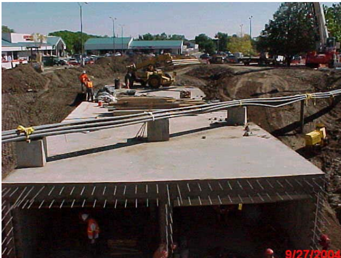
Van Bibber Creek box culvert.
