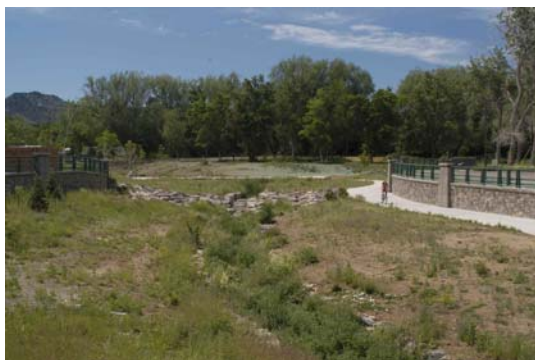
Goose Creek channel, decorative walls and trail
