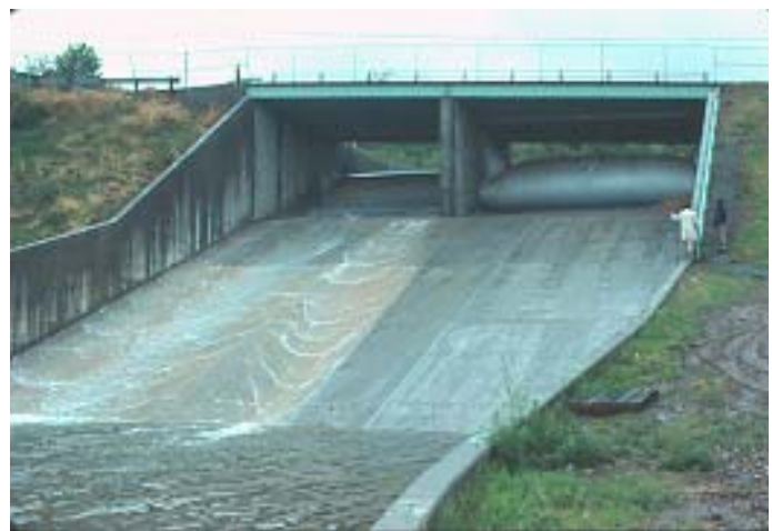
Looking upstream at the old fabridams
