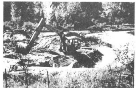
Cleaning out the Willow Creek sediment trap.
