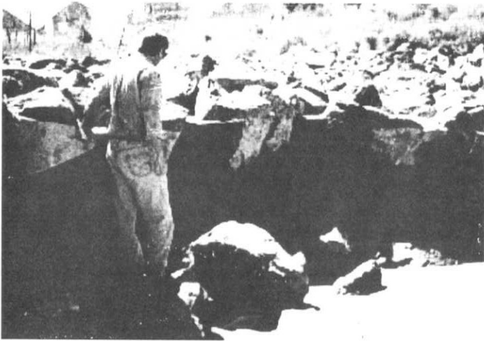
Channel erosion on Sulphur Gulch below the drop structure.
