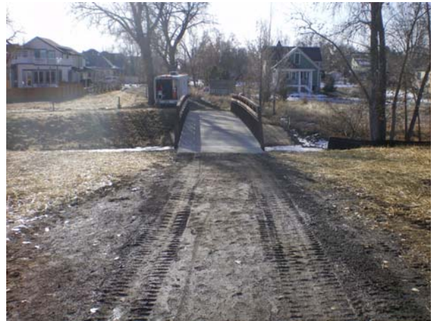
Drainageway #2 pedestrian north of Baseline Road in Lafayette.
