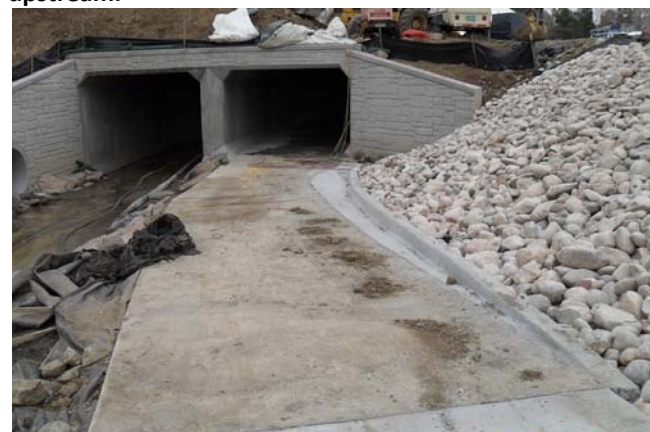
Near Completion – Same view at Arapahoe Road.
