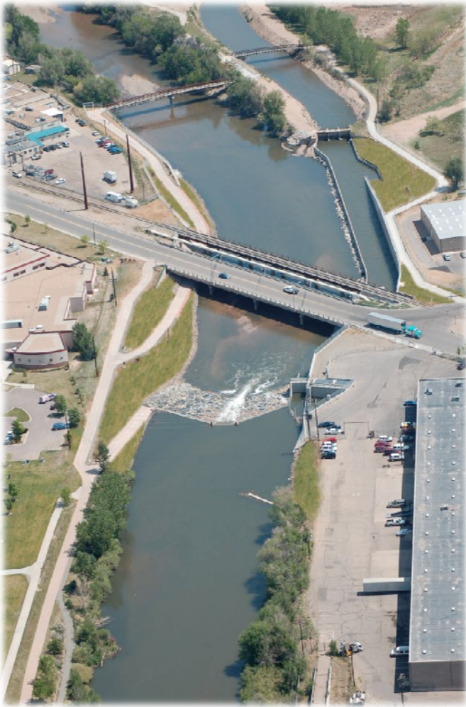
One of the most complex elements of the South Platte River project was the relocated intake structure for the Burlington Ditch (starting below the new traffic bridge on this photo and joining the existing ditch on the top right).
