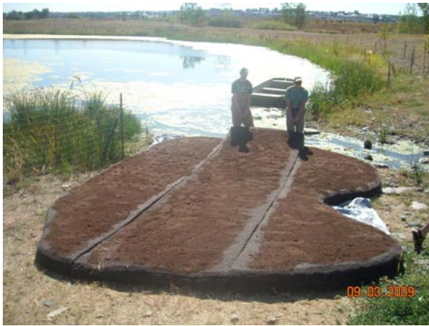
Floating Island during installation
