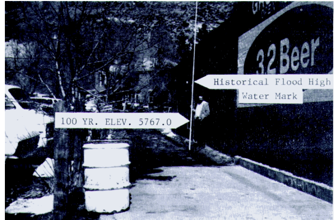
Bear Creek flood levels in Morrison between Market Street and Mount Vernon Street downstream of the Mount Vernon Creek confluence. The “Historical Flood High Water Mark” depicts the level of the September 2, 1938 flood.
