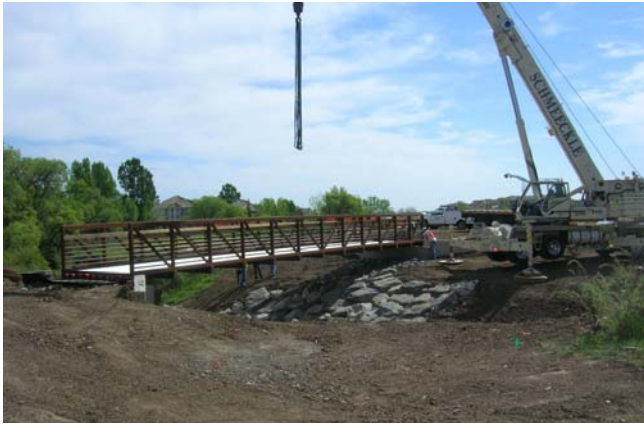
Cottonwood Creek trail construction near Caley Ave and Lima St.
