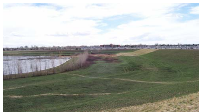
Westerly Creek Dam one month after fire
