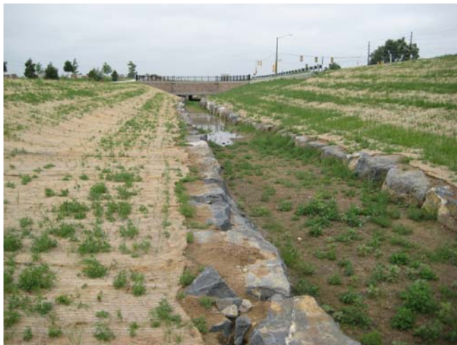
After – City Park Drainageway in Broomfield looking upstream.
