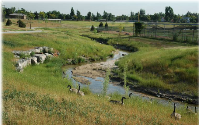
Westerly Creek (what was once in pipe is now returned to the surface).
