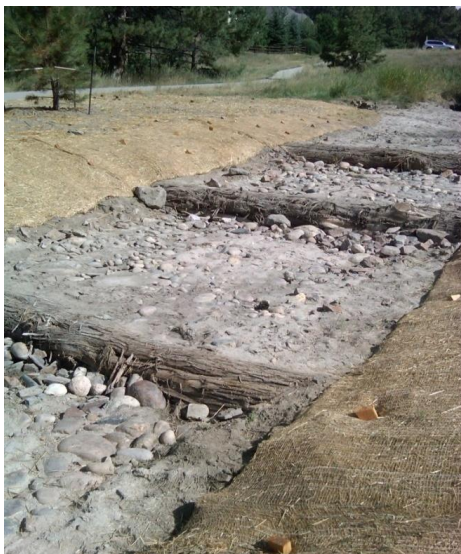
Timber drop structures immediately after construction.
