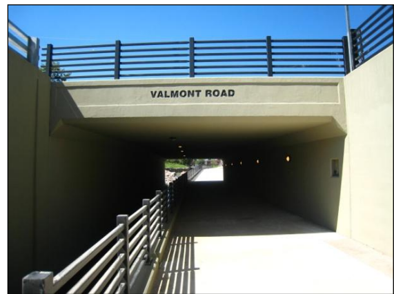
Valmont Road Underpass
