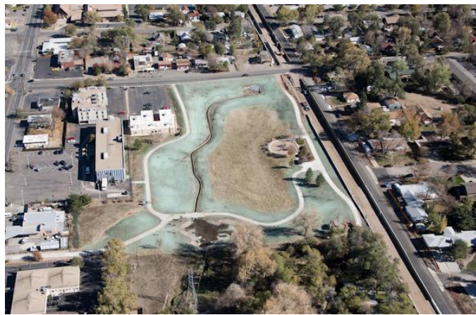
Completed Richey Park detention and water quality improvements. View is looking east with Carr Street in the background and 13 th Avenue and the RTD West Corridor on the right. Photo date is October 29, 2010.
