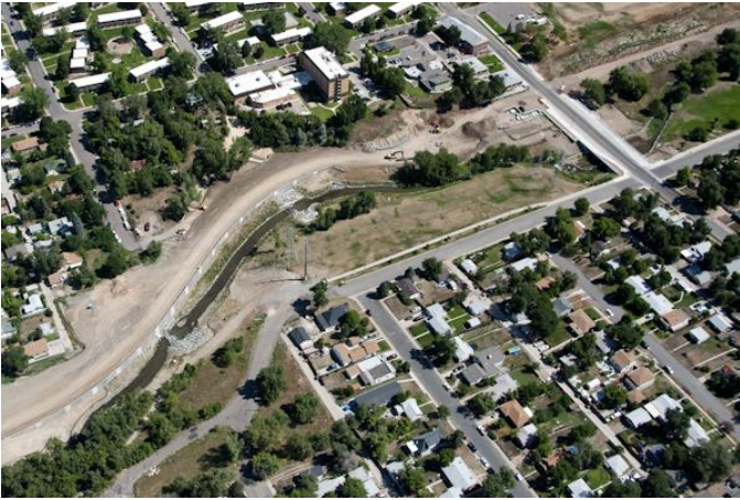
Nearly complete Lakewood Gulch improvements at Knox Court. The Oxbow area is to the north of the West Corridor alignment. View is looking northeast and was taken August 4, 2010.
