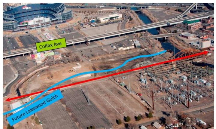
Lower Lakewood Gulch at South Platte River after Decatur Facility Demolition. The future RTD West Corridor Light Rail is in red.
