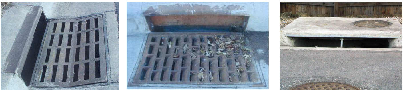
Left to right : CDOT Type 13 grated inlet in combination configuration, Denver No. 16 grated inlet in combination configuration, CDOT Type R curb opening inlet
