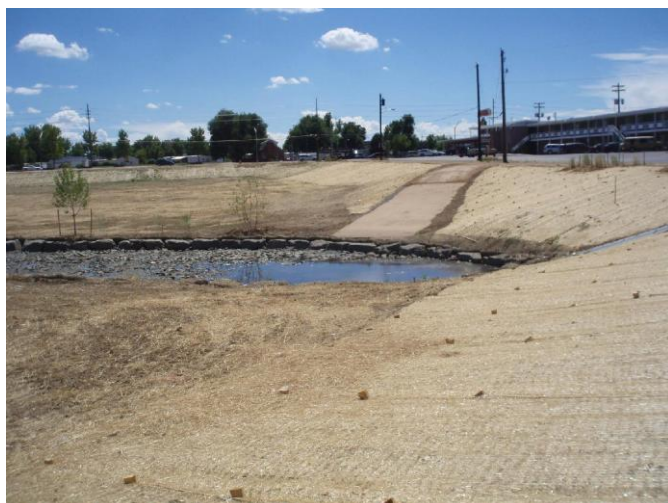
Above, Sable Detention Pond site looking south after construction.
