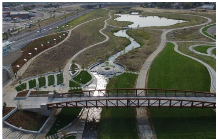
Finished Project Looking East
