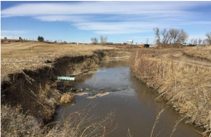
Pre-Construction Looking North
