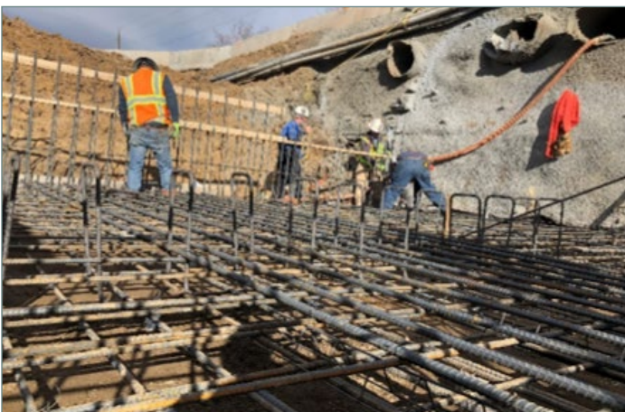
Steel Work on Box Culvert Slab
