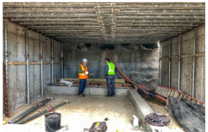
View of Old Culverts and New
