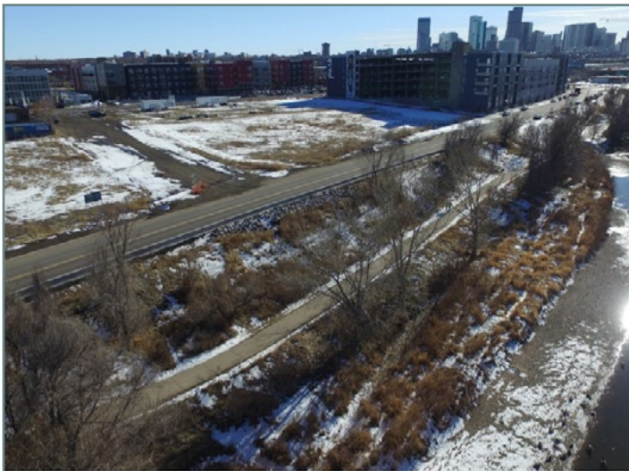
33rd Street Outfall Before
