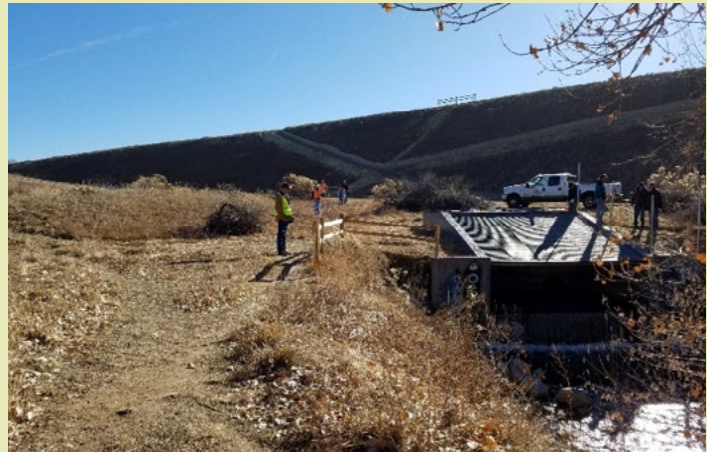
After – Englewood Dam on Willow Creek
