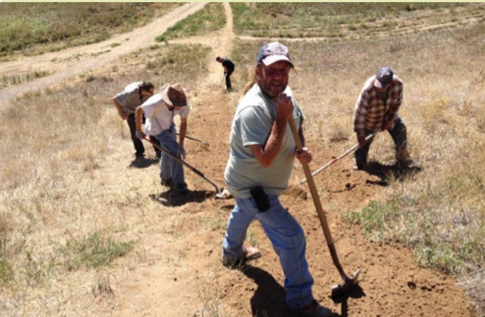
During Construction – Englewood Dam on Willow Creek
