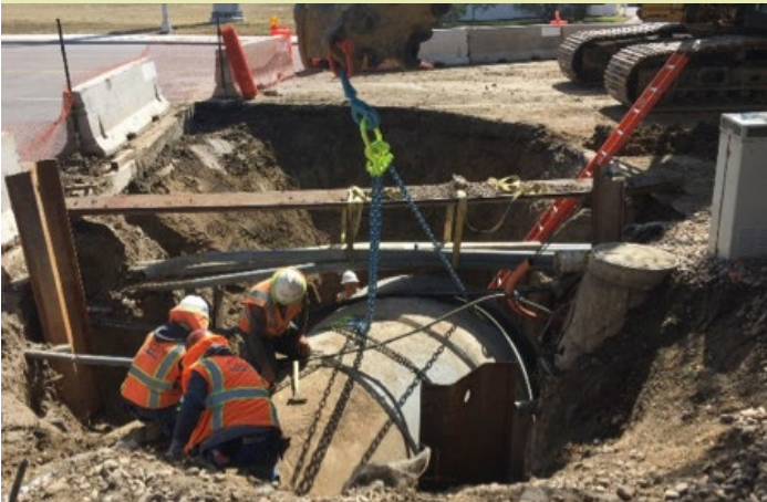
Connecting to the existing 84-inch pipe
