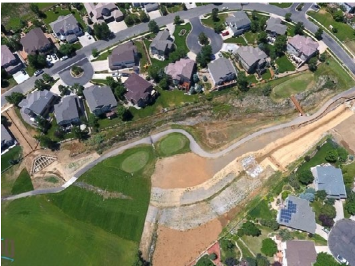
Massey Draw – Oak Street to Rockland Avenue construction completed
