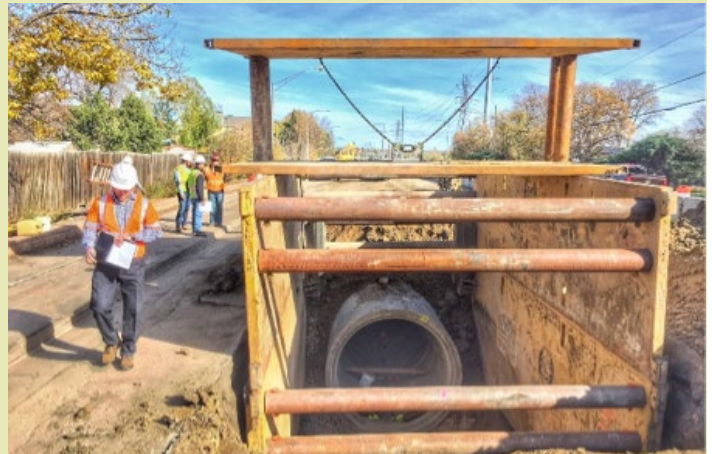
84-inch pipe installation along 88th Ave.
