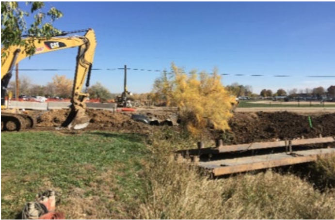
Pre-Construction View of Culvert
