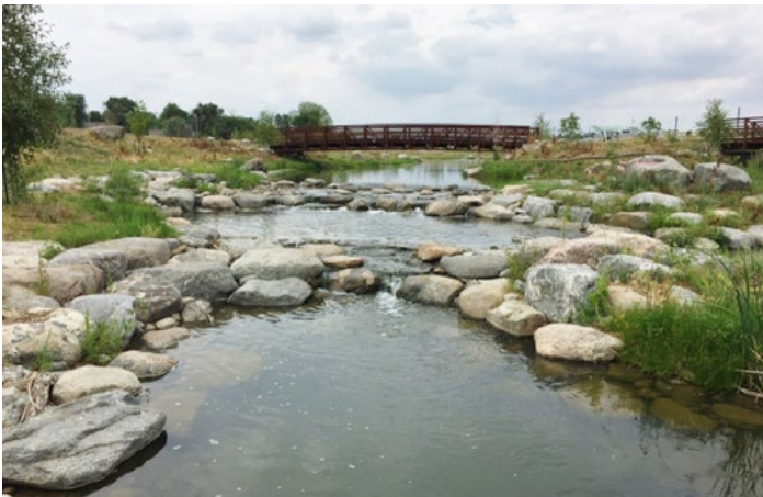
Finished Project at Pond Outlet
