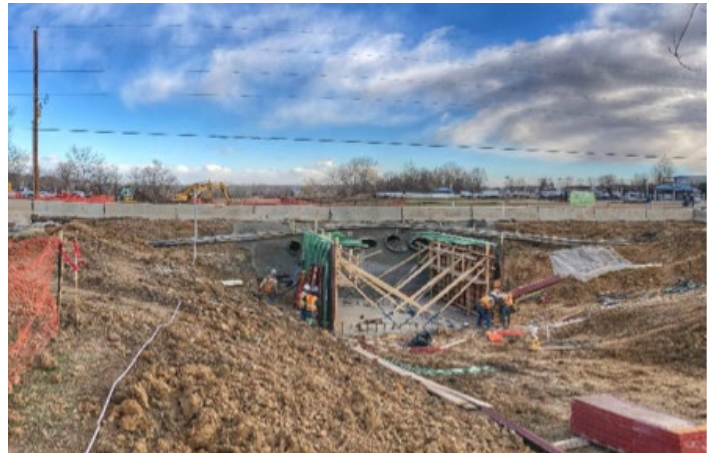
Mid-Construction View of Culvert
