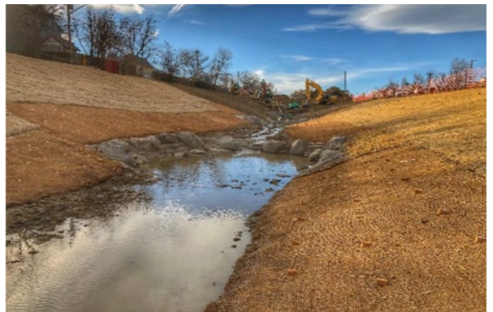
Post-Construction View of Channel
