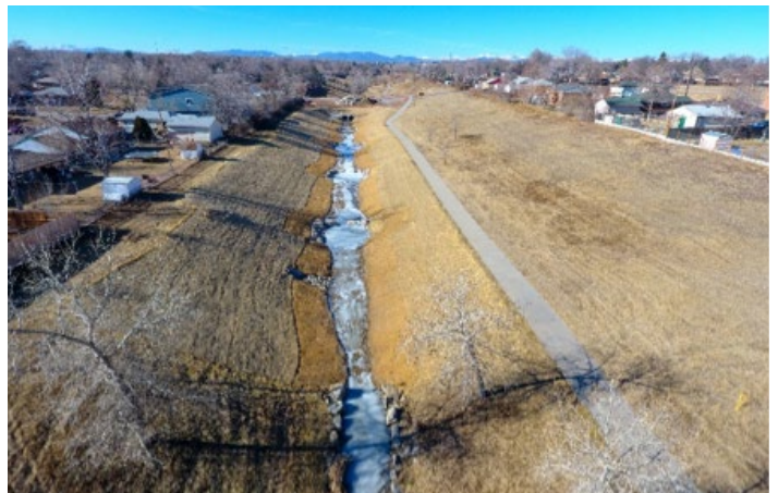
Post-Construction Aerial of Channel
