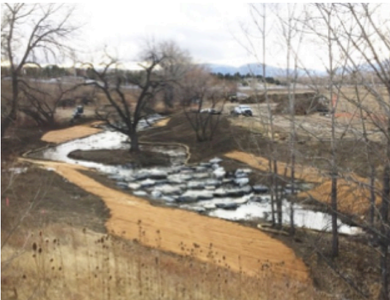
New cascading boulder drop structure on Rock Creek.
