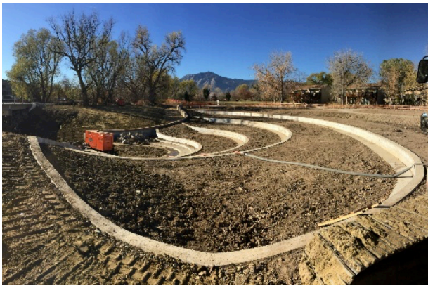
Spillway at the Boulder and White Rock Ditch.
