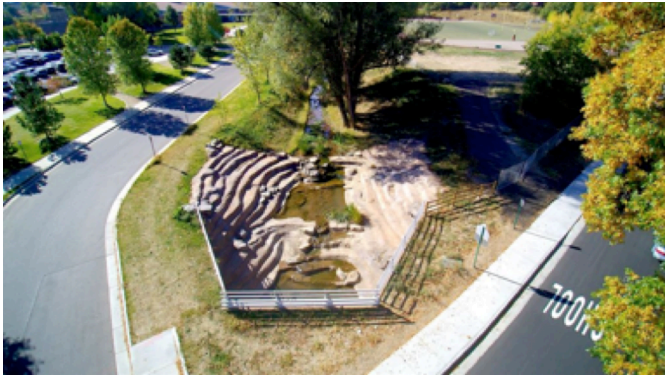
Two-Tier sculpted concrete drop structure on West Fork of Kenney's Run at Golden High School.
