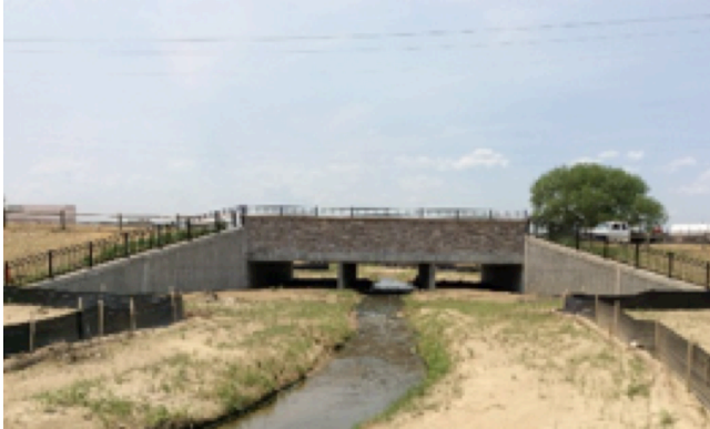
Completed Brantner Gulch crossing structure.
