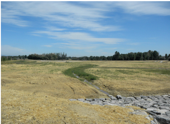
Prince Tributary enters the detention basin over a grouted boulder drop structure protecting the Leyner Cottonwood Ditch.
