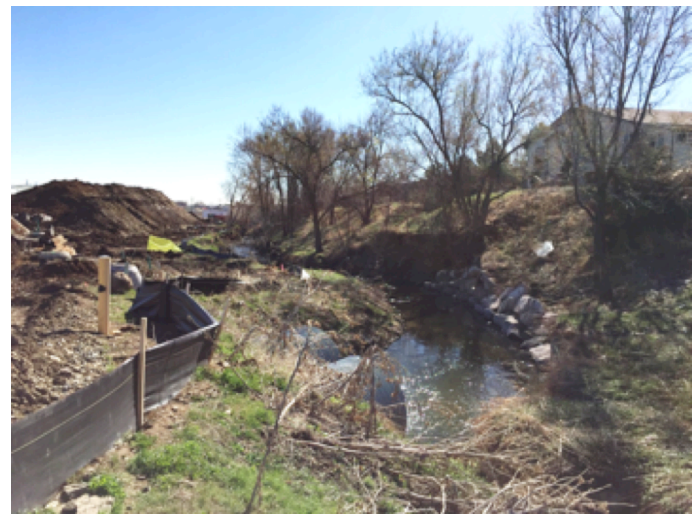
An example of the creek threatening homes.
