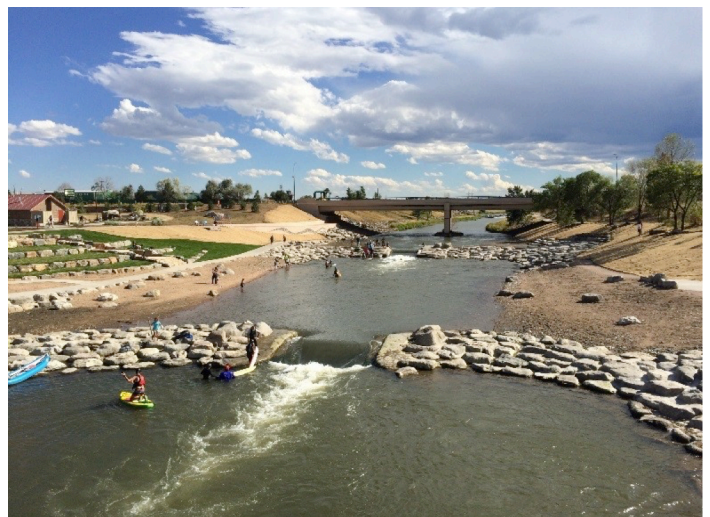
Looking upstream after construction.
