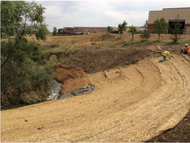
Finished repairs at location two.
