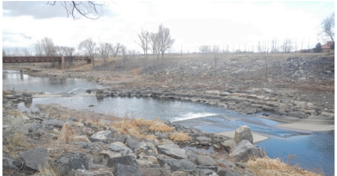
Looking Downstream, Existing Conditions of the South Platte River at Oxford Avenue City of Sheridan, Colorado.
