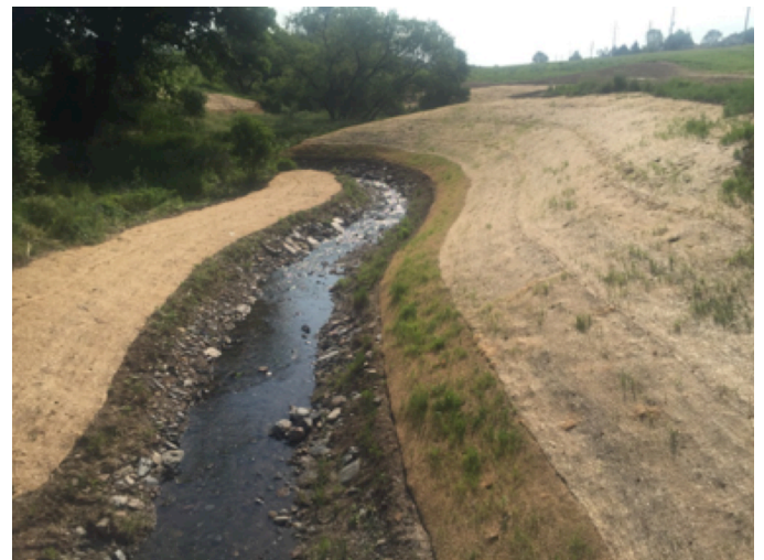
Post-Construction Void-Filled Riprap on Weir Gulch.
