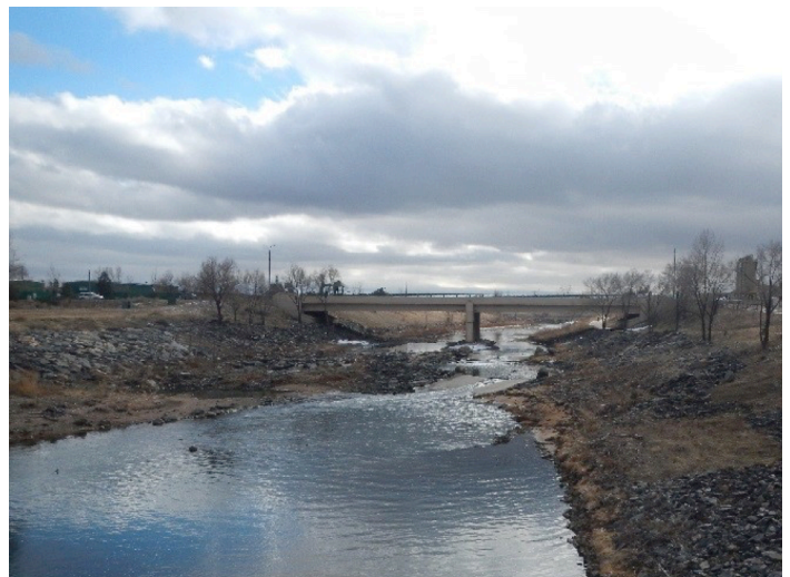
Looking upstream before construction.
