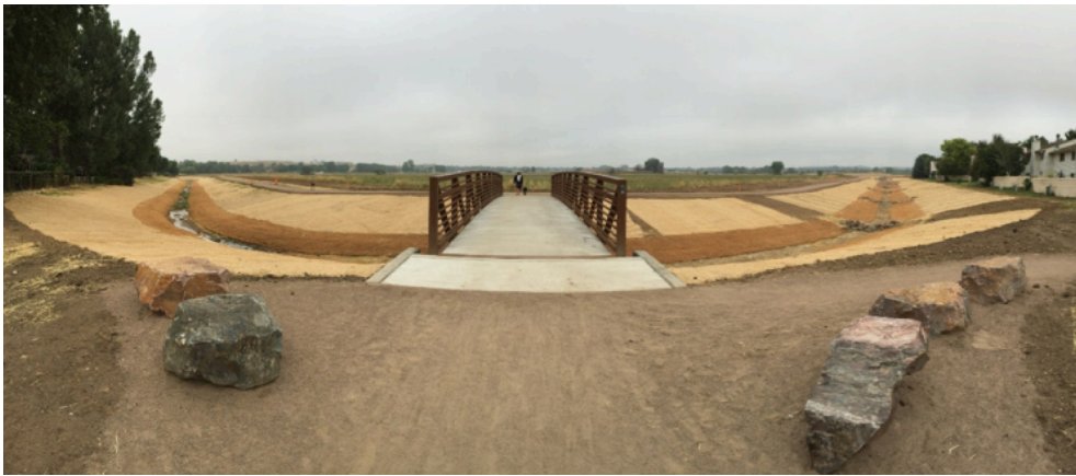
New Pedestrian Crossing and Outfall Channel
