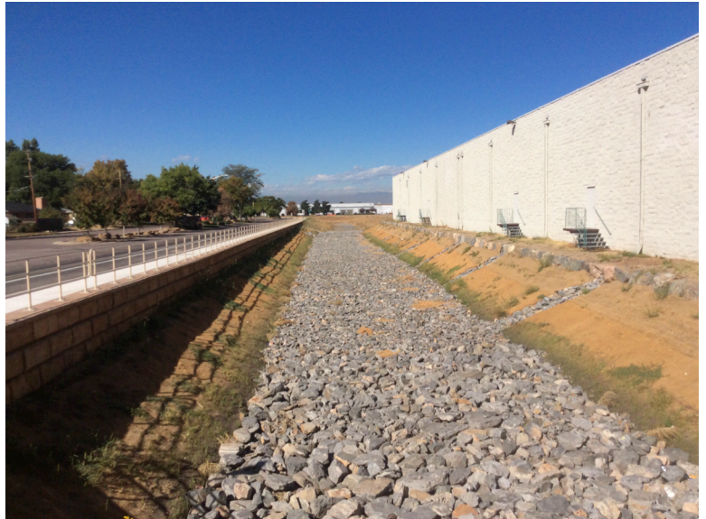
Challenging site constraints with limited right of way for Baranmor Ditch channel improvements. Above-channel before construction; below-improved channel section utilizing block walls to support the added sidewalk on the left and short rock wall on the right to preserve the building access.
