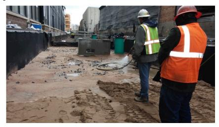
A crew at Industry washes filter media into the structural base of this permeable pavement section. In the distance a second section will be constructed without filter media. Both sections will be monitored for water quality.
