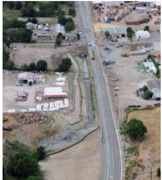
Dry Gulch channel improvements in Lakewood. View is looking west towards Harlan Street. The Light Rail line is bounded by a park and industrial development and adjacent to the channel. The upstream headwall is the confluence of Dry Gulch and North Dry Gulch. This photo was taken on September 12, 2011.
