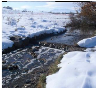
Completed timber drop
