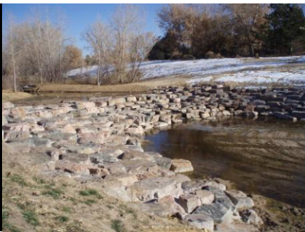
The check structures were turned into drop structures (left) and the channel was reshaped (center and right)
