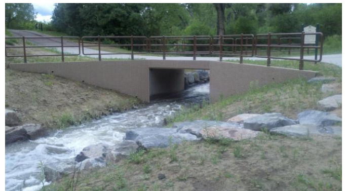
Lee Gulch at the High Line Canal after construction
