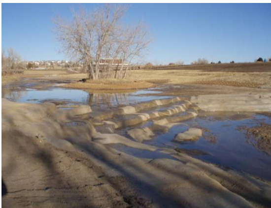
Two sculpted drop structures were also constructed
