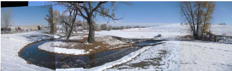
Post-construction view of concrete log drop and bio-logs
