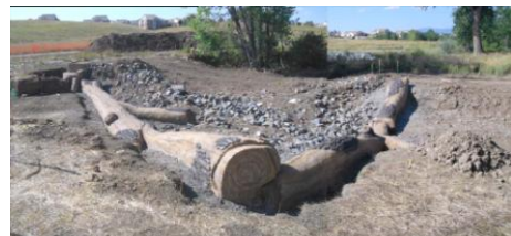
Concrete log drop during construction
