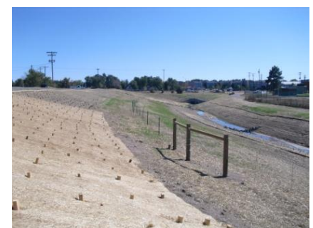
North Outfall pipeline construction and finished outfall channel
