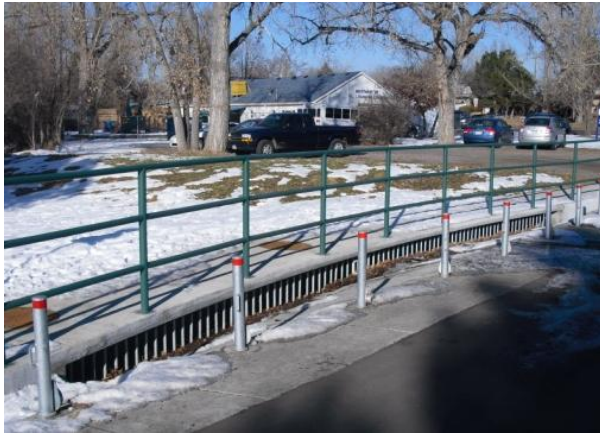
Shaw Heights Tributary completed 45-foot special curb inlet
