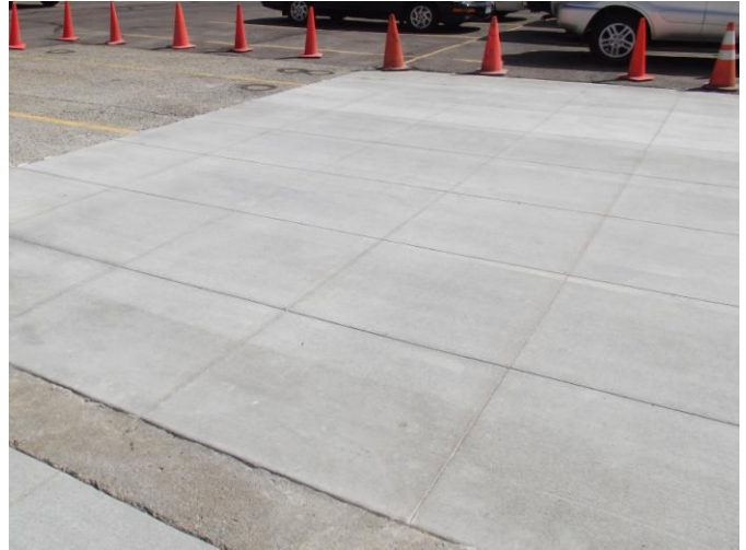
New permeable pavement test pad in Lakewood
