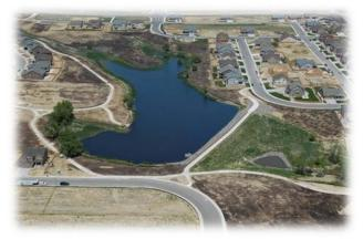
Marshall Lake Dam, flood control was provided above the permanent water surface as a result of dam rehabilitation under the supervision of State Engineer's Office. Horizon Tributary to Brantner Gulch was stabilized throughout this development. 136<sup>th</sup> Avenue is visible in the background.
