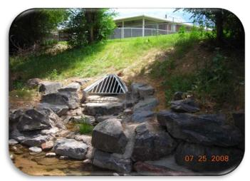
The 36-inch storm sewer outlet to Big Dry Creek is protected from erosion with grouted boulders
