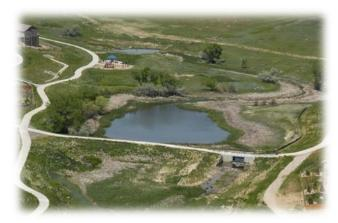
Villages at Riverdale regional water quality pond. An existing agricultural pond was rehabilitated with a new water quality outlet structure and discharge pipe, embankment repairs and high level outlet control. The trail crossing is above the 10-year water surface, more infrequent discharges overtop the trail. The forebay is visible upper-left. The area between the forebay and dam embankment was not disturbed.
