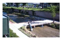
performed the survey and estimated that the peak flow was at least 4,100 cfs. This discharge equals the 10-year flood
