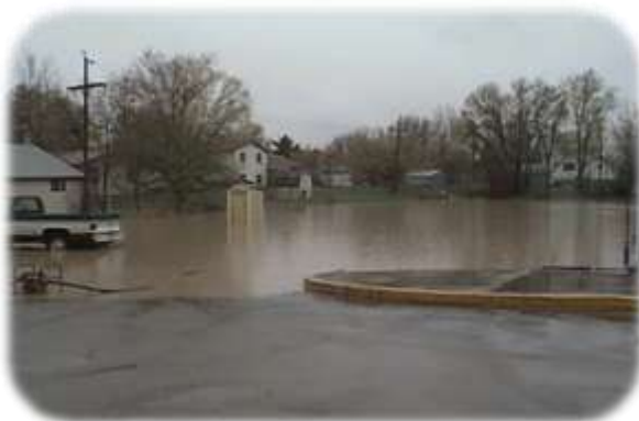
Flooding along Tributary CC-10-in Erie.
