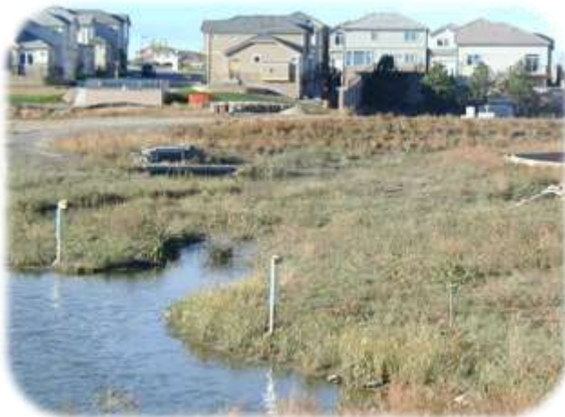
Cottonwood Creek at Peoria Street, a water quality pond which doubles as a wildlife sanctuary. The bird houses on poles are actually indicators of the sediment level in the pond and outline the hidden maintenance access road.
