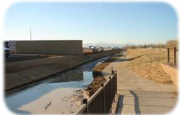
Channel constructed to control flooding shown at left.
