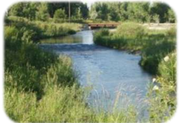
Main channel with low flow crossing and riffle drop
