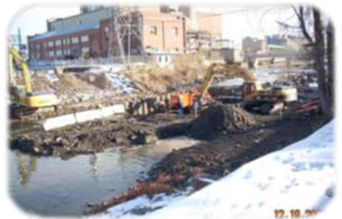
Zuni/Sun Valley Reach - Utility Work Downstream of 13 th Avenue
