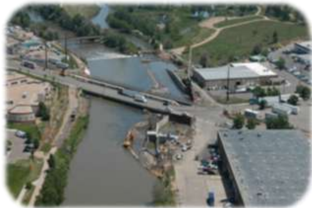
Channel Construction in Globeville at Franklin Street
