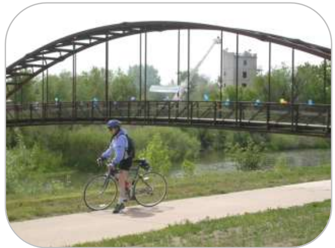
Big Dry Creek Trail Bridge at the Confluence with the South Platte River
