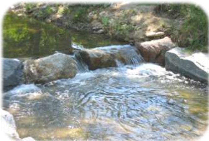
Rock Drop Structure near Broadway
