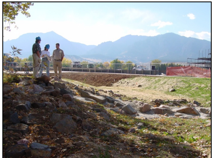
Private development construction inspection for UDFCD maintenance eligibility
