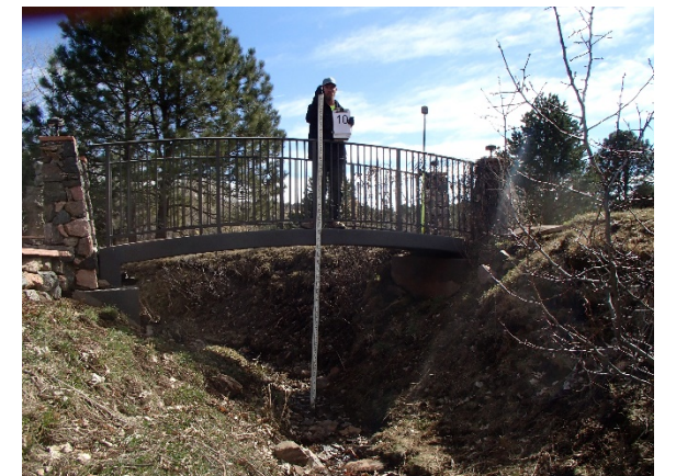
Reach WC-5: Structure 10 – Pedestrian Bridge 13-ft Bridge (no piers)
