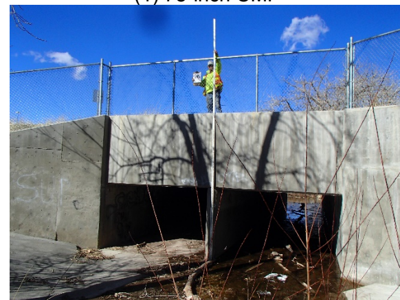
Reach WC-4: Structure 26 – Eldridge Street (2) 10-ft by 6-ft RCBC
