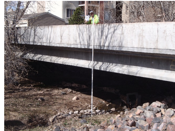
Reach WC-2: Structure 37 – Pedestrian Bridge 90-ft Bridge (no piers)
