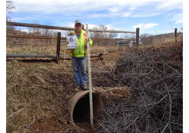
Reach WC-5: Structure 6 – W. Roton Arena (1) 36-inch RCP
