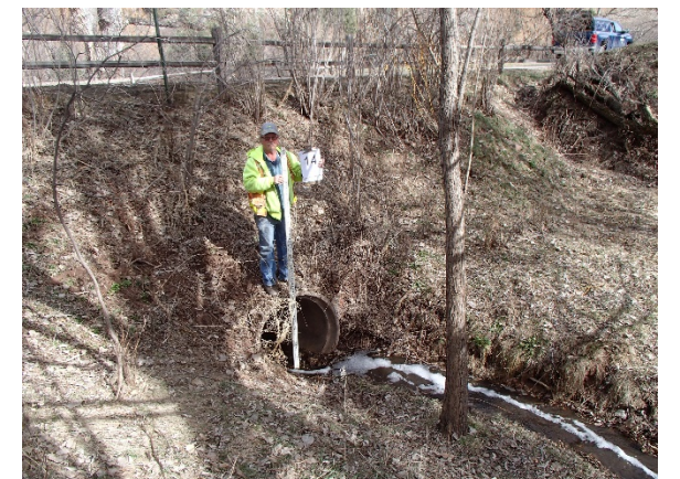
Reach WC-5: Structure 14 – Willowbrook Drive (1) 36-inch RCP
