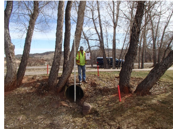
Reach WC-5: Structure 4 – Golf Cart Path (1) 24-inch ABS, (1) 36-inch Steel Pipe
