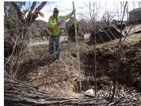
Reach WC-5: Structure 9 – Private Driveway (1) 32-inch by 28-inch Elliptical CMP
