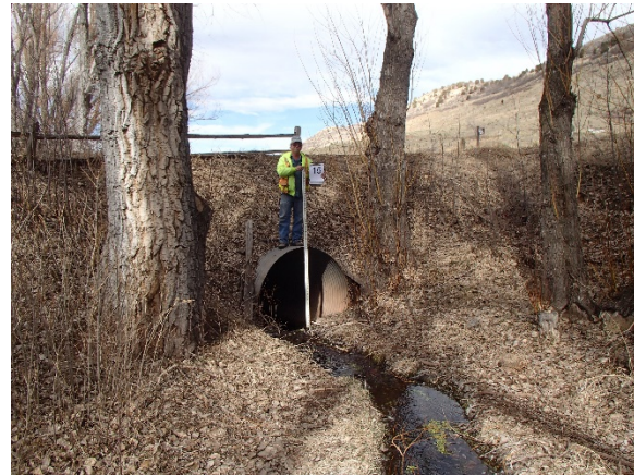
Reach WC-5: Structure 15 – Crestbrook Drive (1) 72-inch CMP
