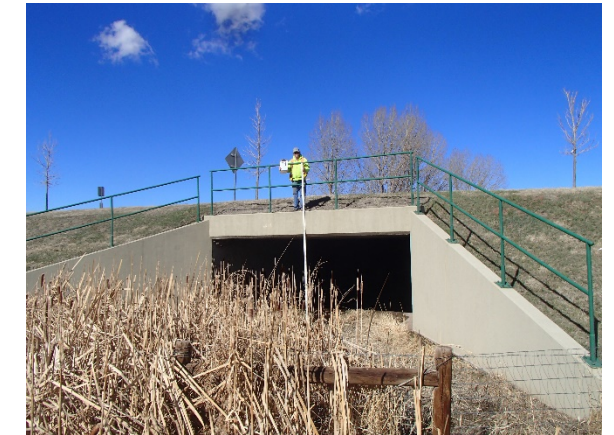
Reach WC-5: Structure 24 – Quincy Avenue/Frontage Road (1) 20-ft by 8-ft RCBC
