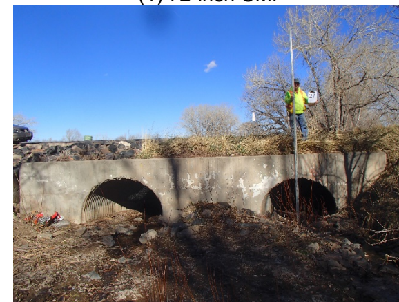
Reach WC-4: Structure 27 – Cole Street (2) 68-inch CMP
