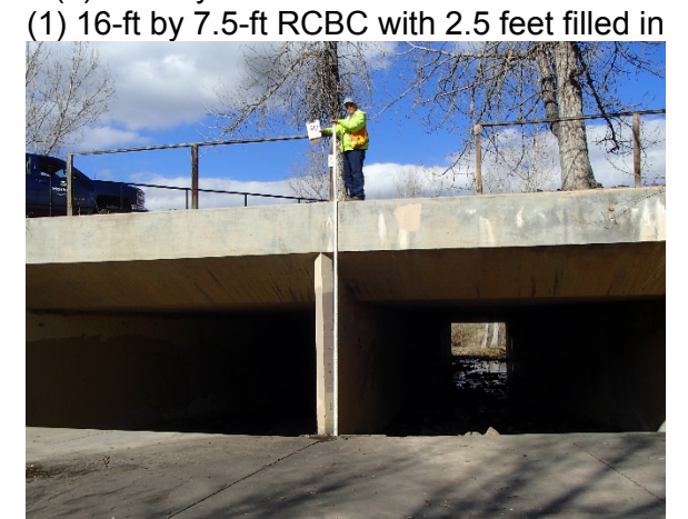
Reach WC-1: Structure 40 – Dartmouth Avenue (2) 22.5-ft by 9.2-ft RCBC (Modified Drop Inlet) (14-ft by 9.2-ft RCBC at Throat)
