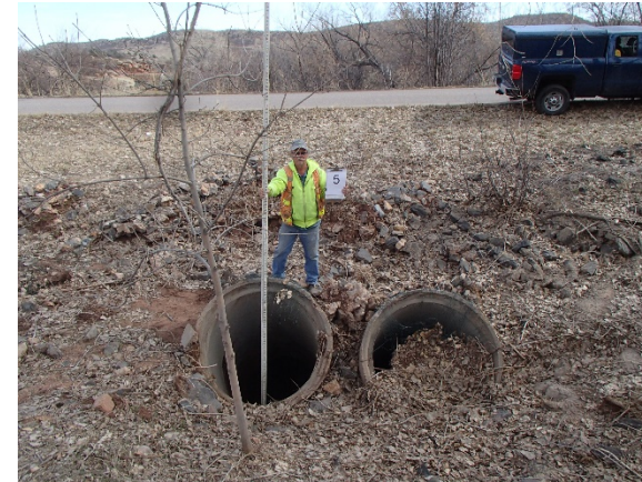
Reach WC-5: Structure 5 – Willow Springs Drive (2) 48-inch RCP (Modified Drop Inlet)
