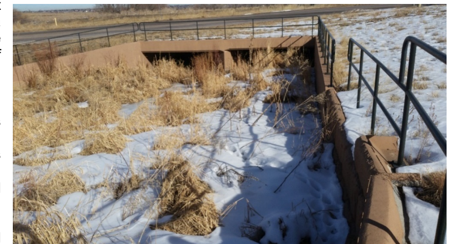
Photo 3: MDP Reach WC-3 – Existing Crossing Underneath Quincy Avenue
