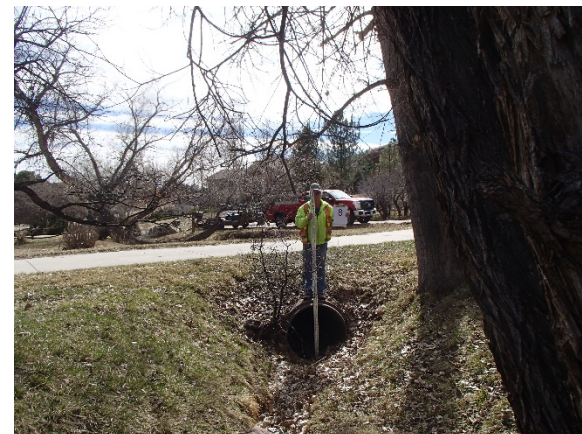
Reach WC-5: Structure 8 – Private Driveway (1) 36-inch RCP
