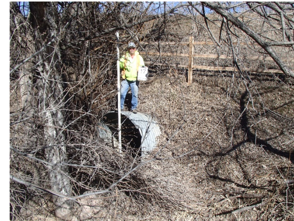
Reach WC-5: Structure 17 – Belleview Avenue (1) 72-inch CMP
