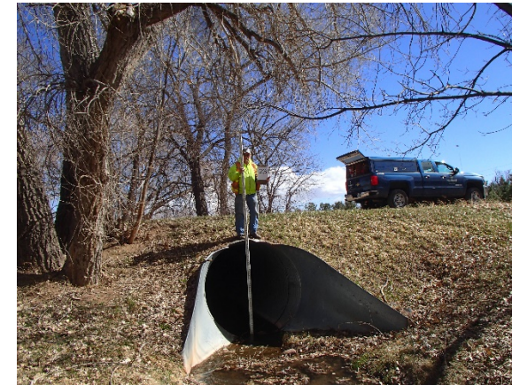
Reach WC-5: Structure 23 – Private Driveway (1) 72-inch CMP
