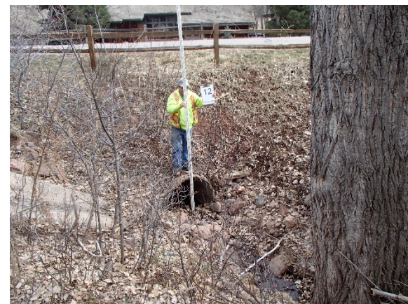
Reach WC-5: Structure 12 – Colorow Drive (1) 36-inch RCP
