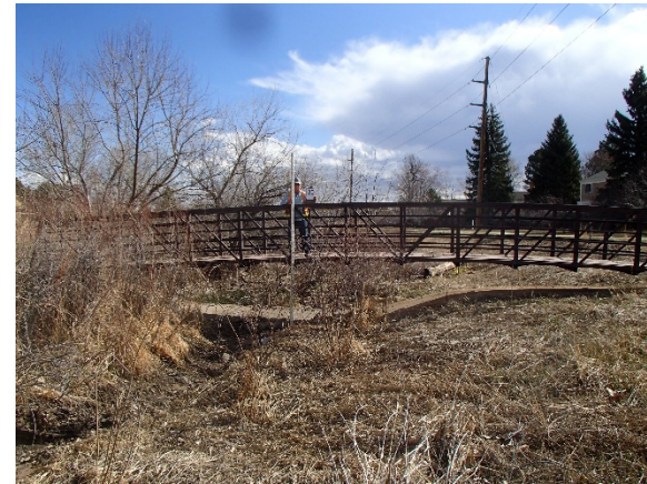
Reach WC-3: Structure 30 – Pedestrian Bridge 60-ft Bridge (no piers)
