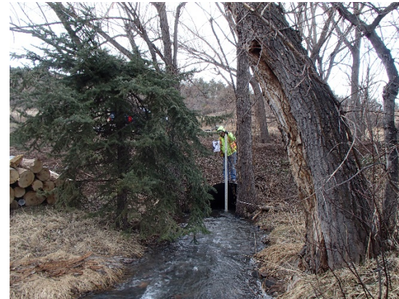
Reach WC-5: Structure 16 – Private Driveway (1) 6-ft by 3.7-ft Elliptical CMP
