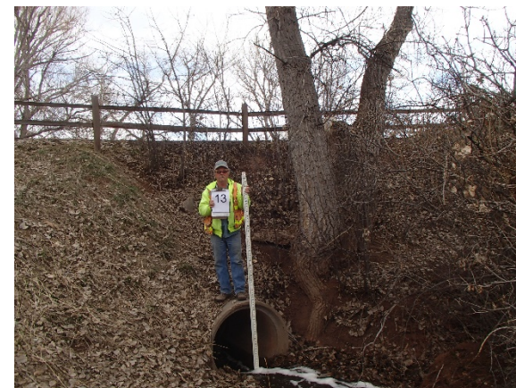
Reach WC-5: Structure 13 – Meadowbrook Drive (1) 36-inch RCP
