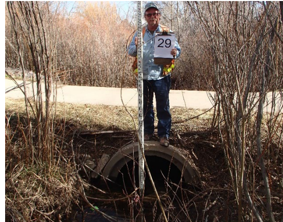
Reach WC-4: Structure 29 – Pedestrian Walkway (1) 36-inch RCP
