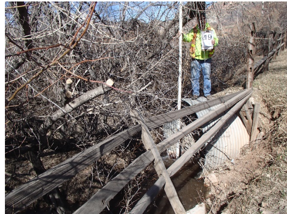
Reach WC-5: Structure 19 – Belleview Avenue (1) 74-inch CMP
