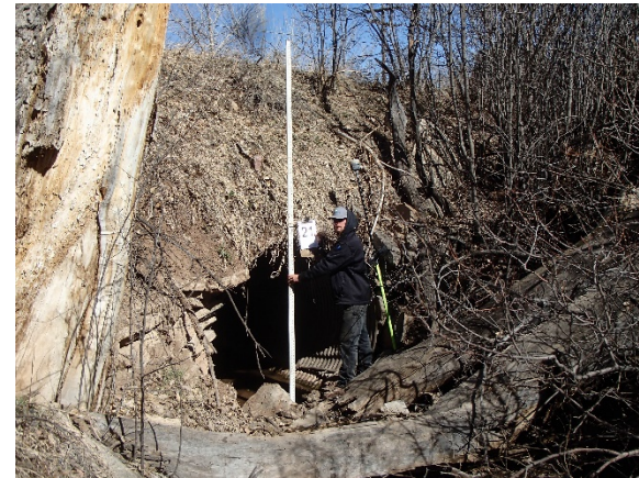
Reach WC-5: Structure 21 – Belleview Avenue (1) 78-inch CMP
