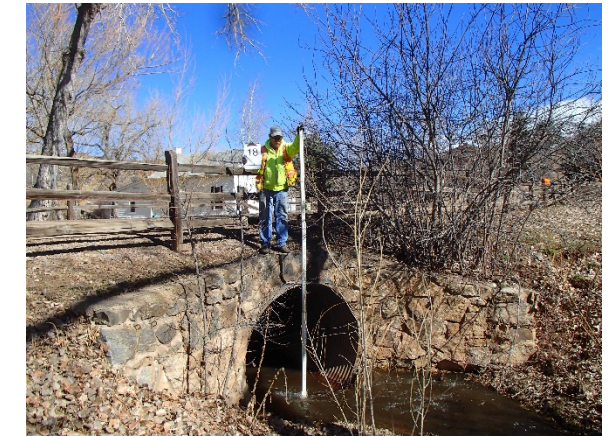
Reach WC-5: Structure 18 – Private Driveway (1) 72-inch CMP
