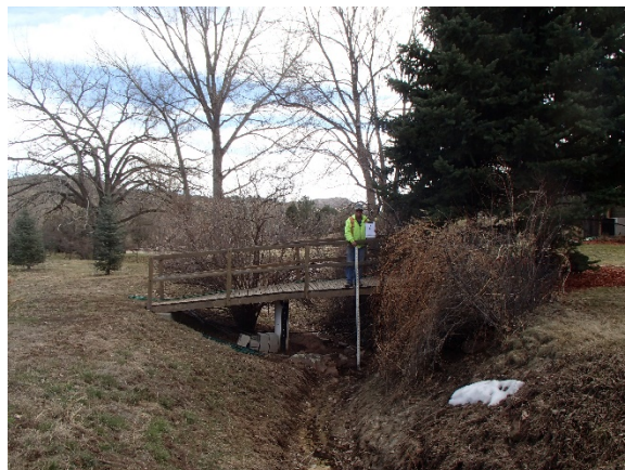
Reach WC-5: Structure 7 – Pedestrian Bridge 19.5-ft Bridge (1 pier)
