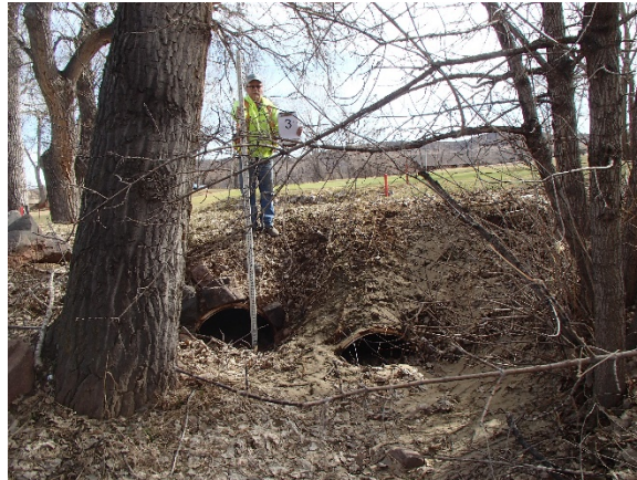
Reach WC-5: Structure 3 – Golf Cart Path (2) 36-inch Steel Pipe
