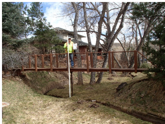
Reach WC-5: Structure 11 – Pedestrian Bridge 29.5-ft Bridge (1 pier)
