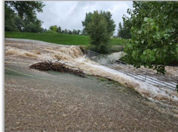
August 16, 2022, Storm Damage:
