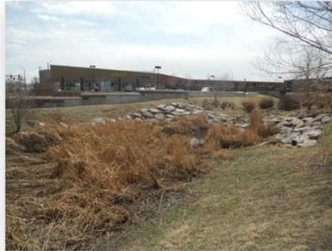
Channelized portion of North Dry Gulch at Walmart Business Park
