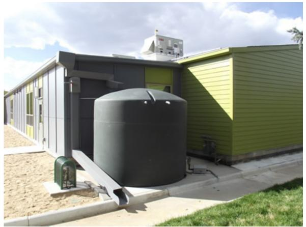
The 3000 gallon cistern collects runoff from approximately 7300 square feet of the roof. The purge valve is shown at the lower right side of the cistern. This box includes a pressure transducer continuously measuring the volume in the cistern. A valve on the downspout allows for winterizing the system. A rain gauge can be seen mounted on the HVAC box.
