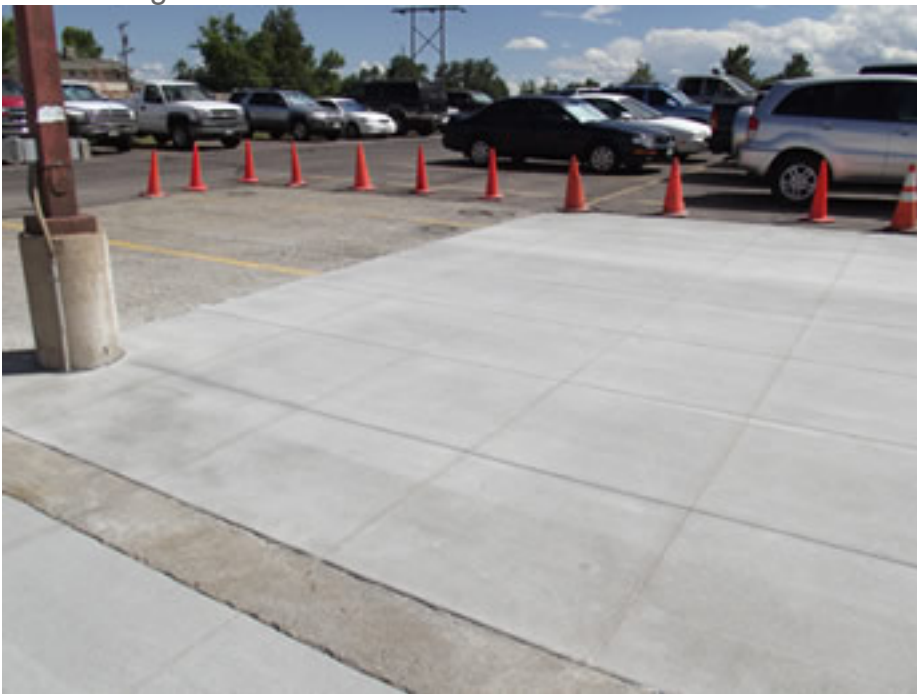
Slotted concrete following construction in 2011.
