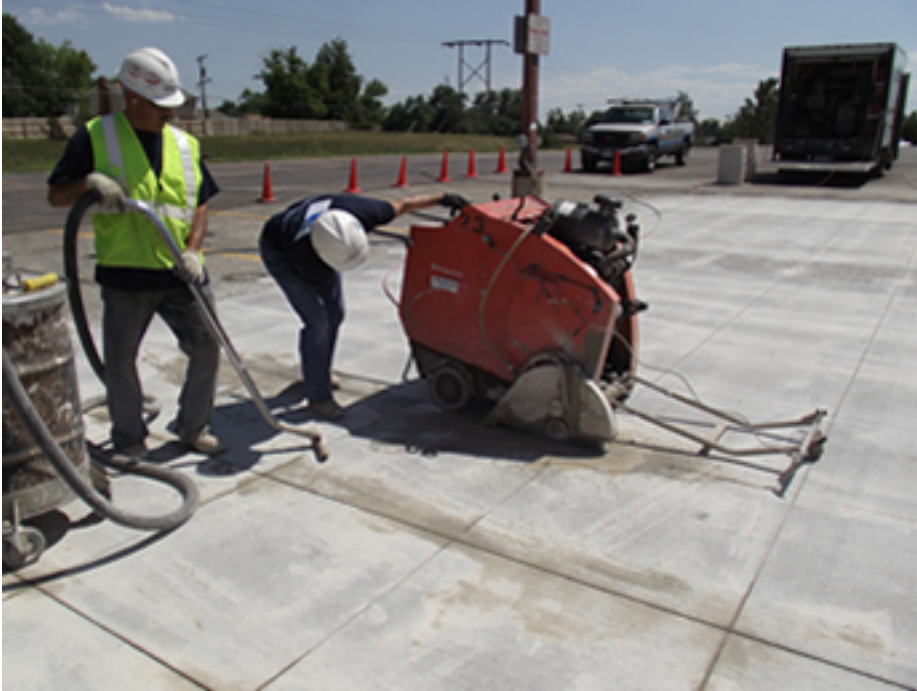
Saw cutting slotted concrete.
