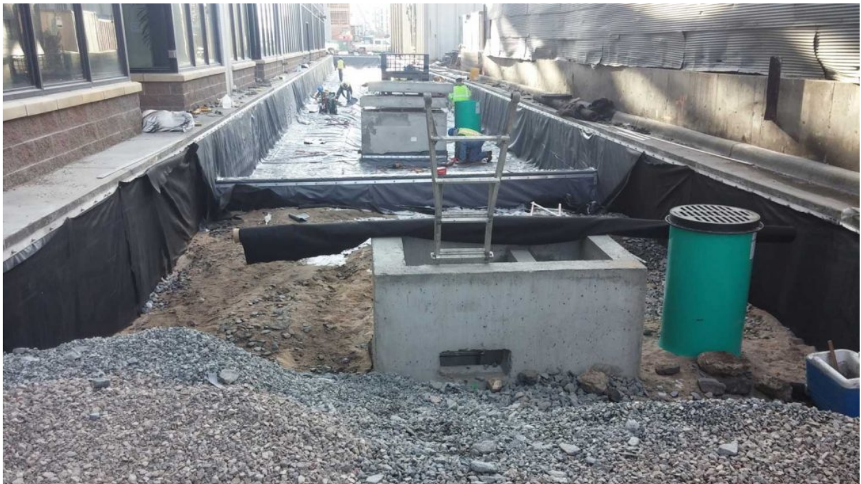
Sections 1 and 2 are separated by a concrete wall
